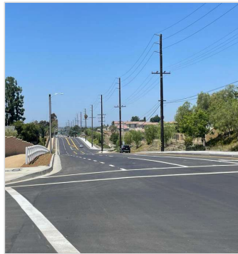
Bastanchury Road Improvements City of Yorba Linda
