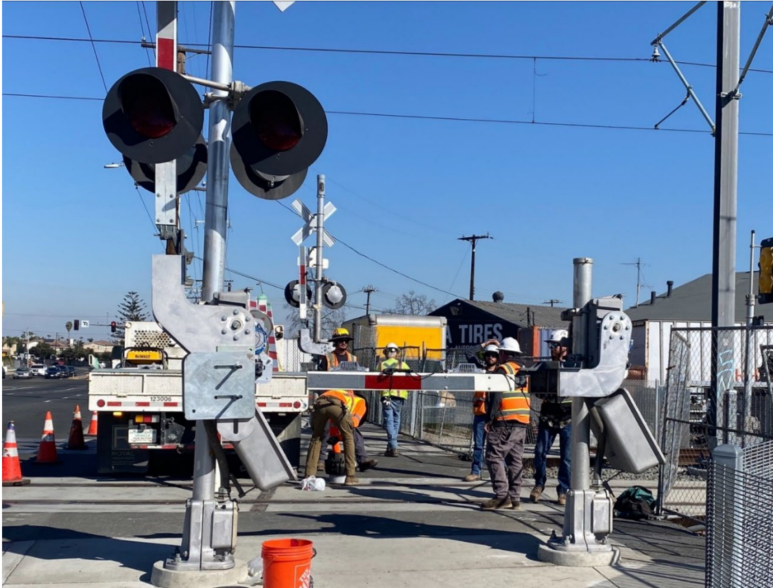
Fairview Street crossing signal and train control installation
