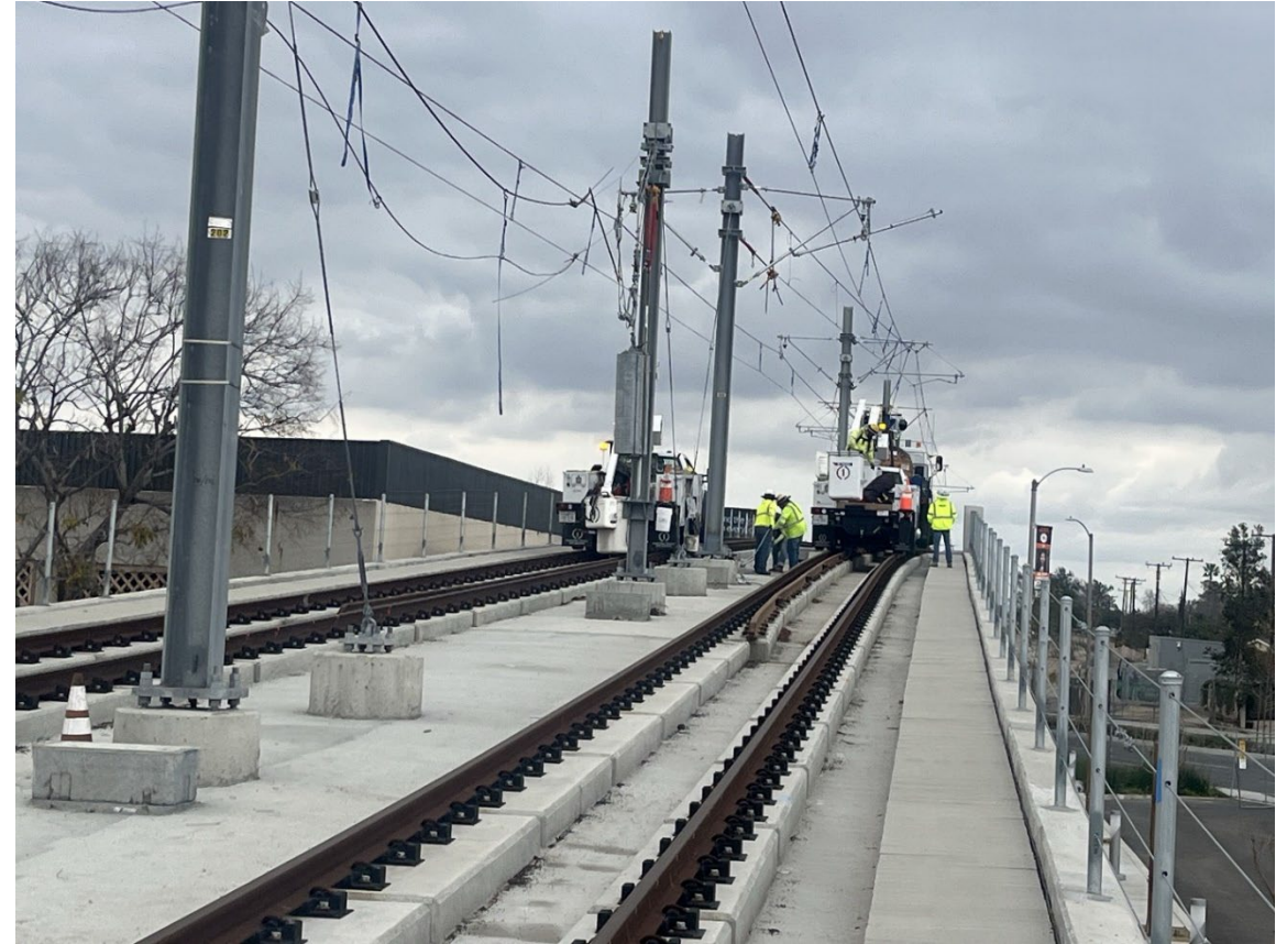
Overhead contact system work at Westminster Avenue bridge
