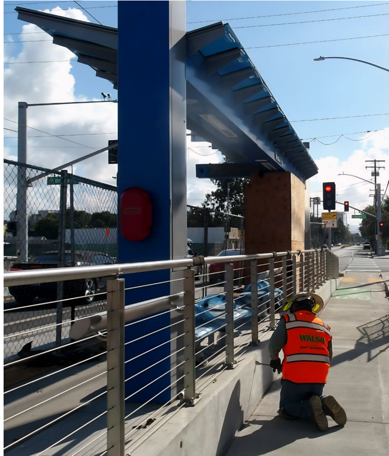
Bristol Street platform punchlist work
