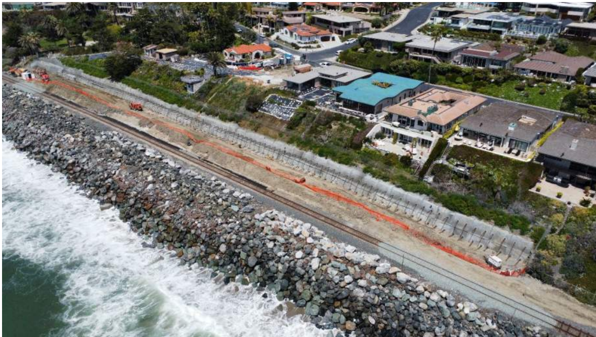
Figure 1 MP 206.80 Track Stabilization Project (Cyprus Shore) May 2023
