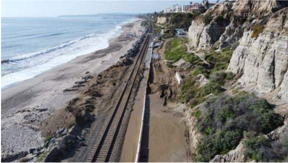
Figure 10. Monitoring Site #6: MP 206.10, Calafia State Beach, January 2024
