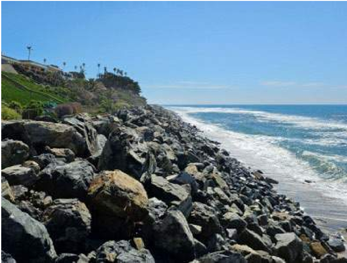
Figure 11. Monitoring Site 7: MP 206.70–207.25, Cyprus Shore to County Line, December 2023
