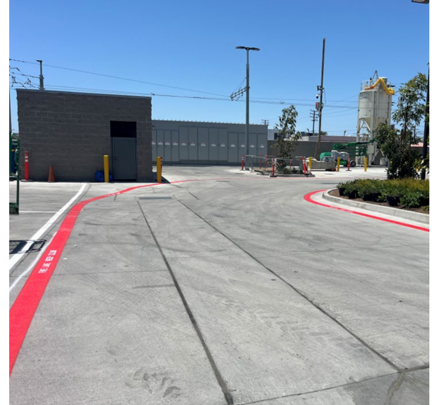
Parking lot striping, including fire lane
