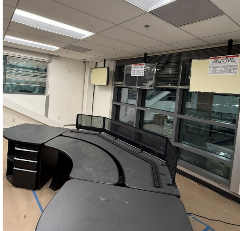
Installation of furniture and workstations
