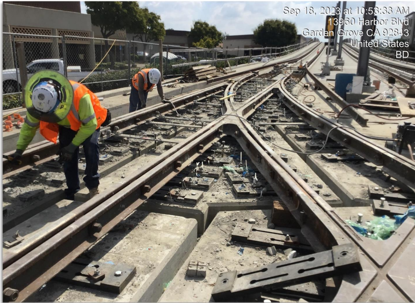
Double Cross-Over and Train Signal at Harbor Station
