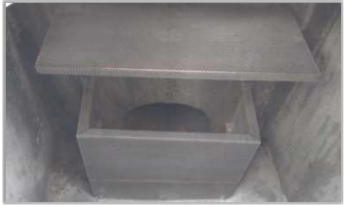
Connector Pipe Screen
