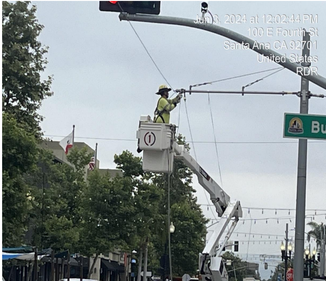
Installation of OCS Bracket Arms
