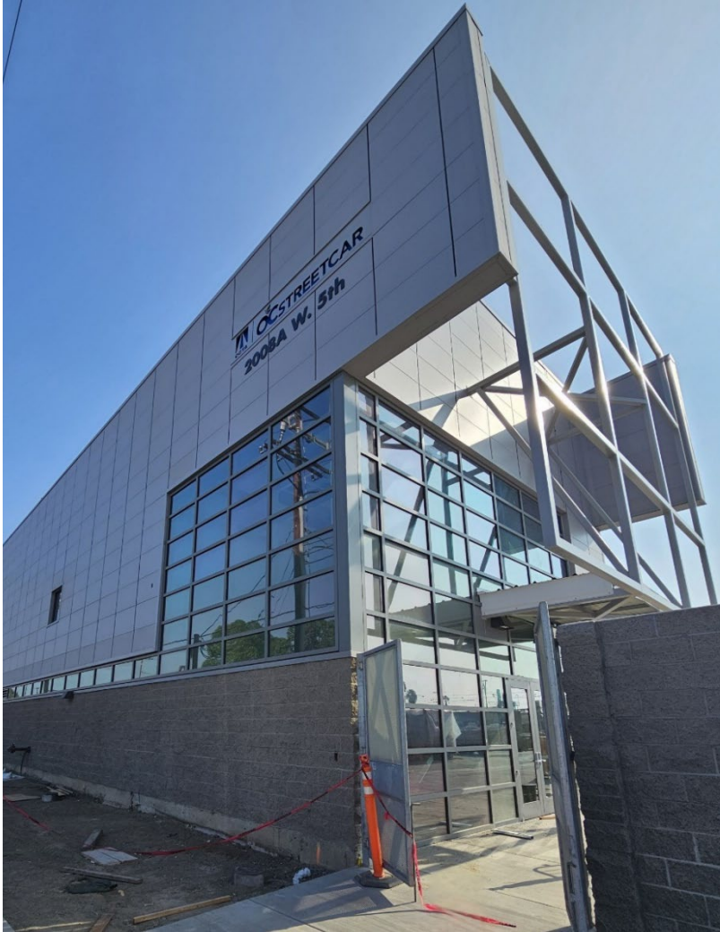
Installed Building Signage
