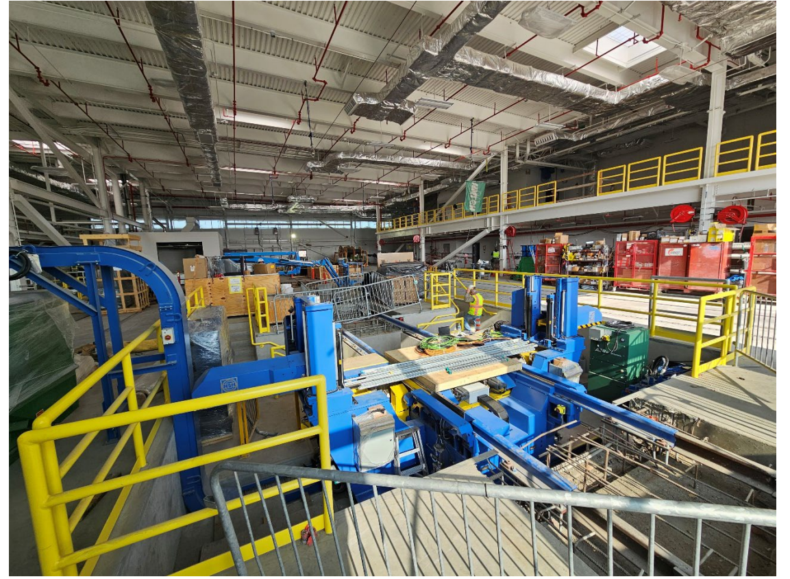
Interior of MSF
