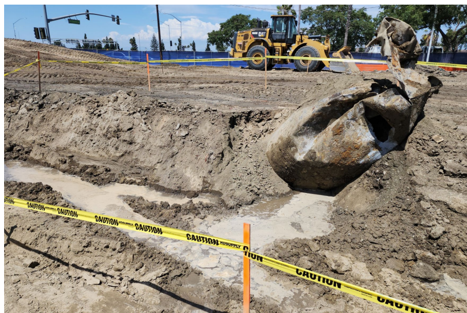
Underground storage tank (UST) 1
