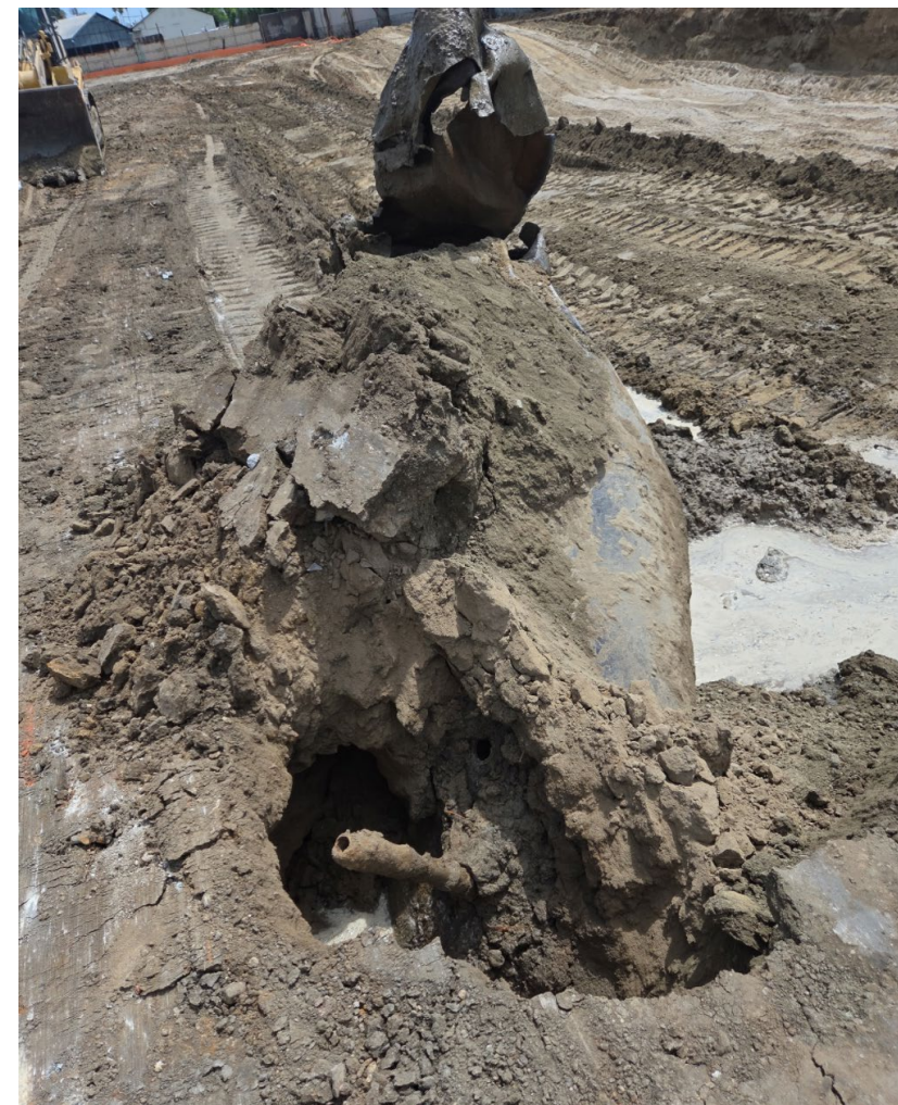
Underground storage tank (UST) 1
