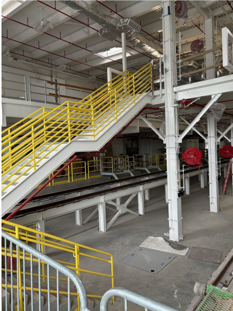
Maintenance Bay No. 1
