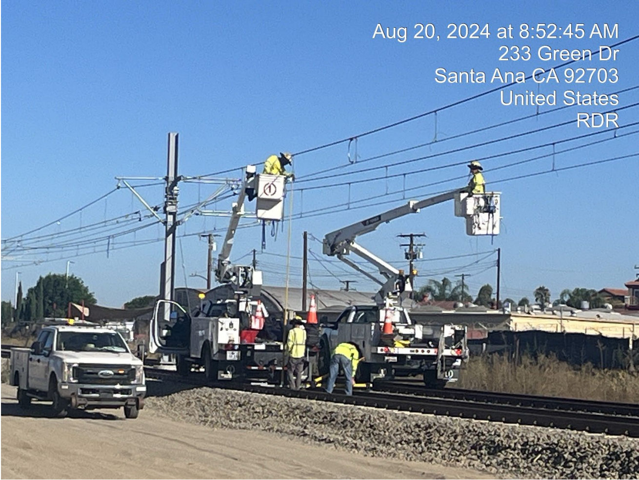
Overhead contact system (OCS) wire installation
