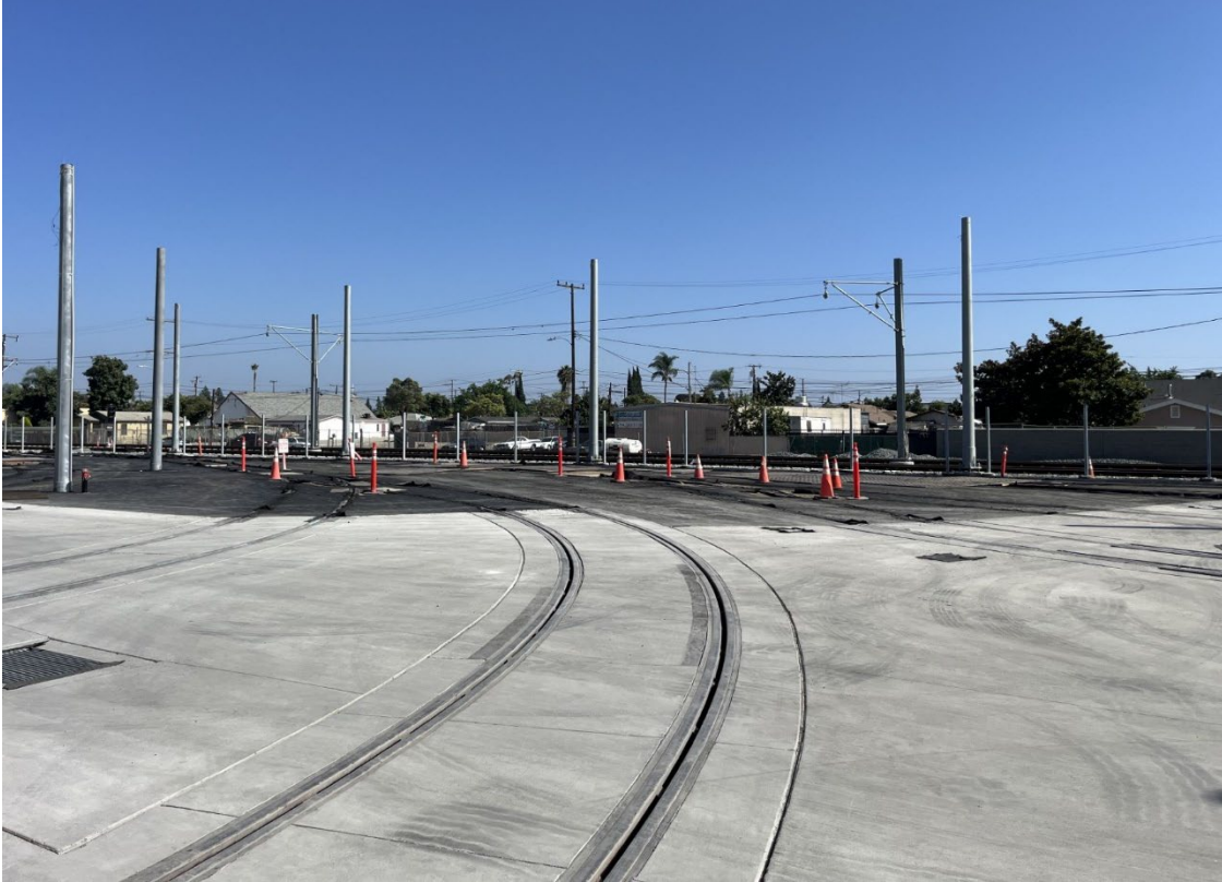
Yard track paving
