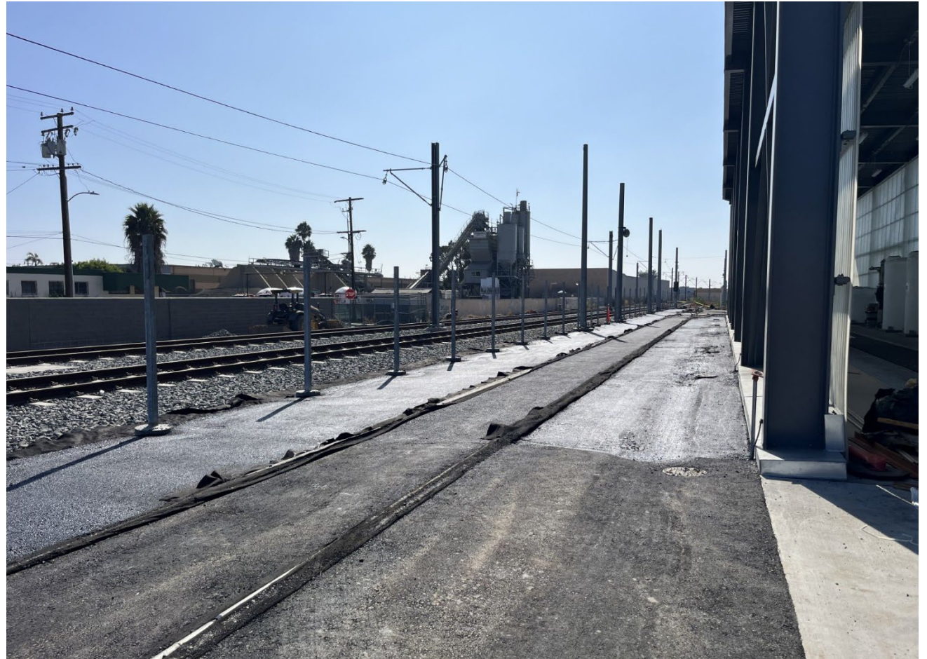
Paving behind car wash
