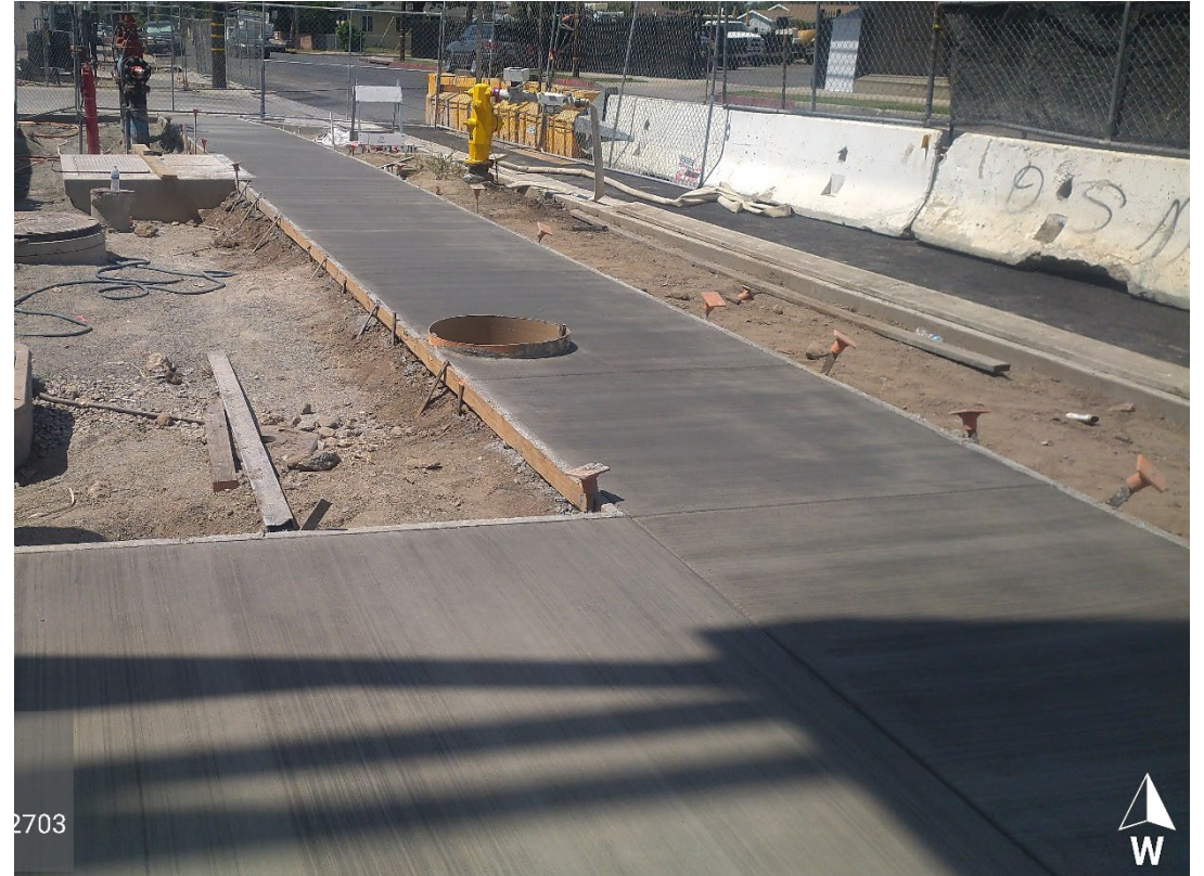
Sidewalk along Fifth Street
