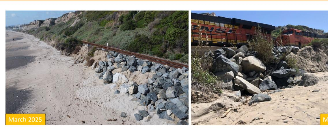
Area 4 - Eroding Embankment and Degrading Riprap Adjacent to Active Track
