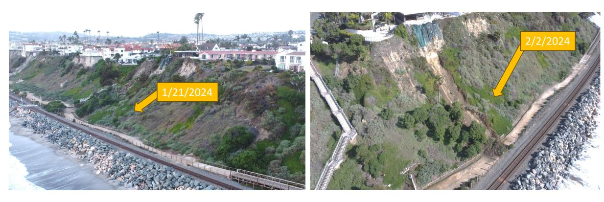
Area 3 - Landslides Adjacent to Active Track North of Pedestrian Bridge
