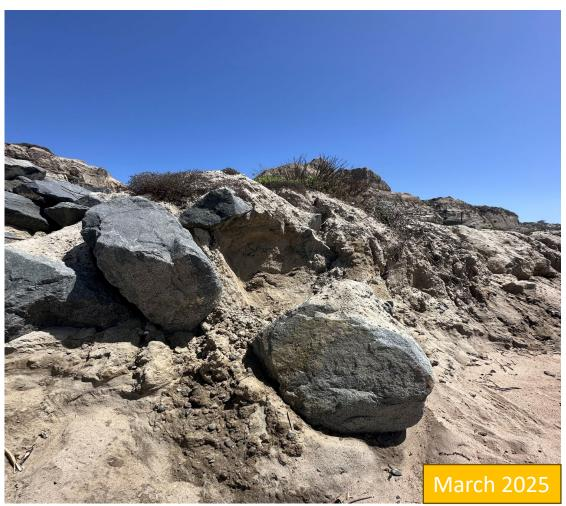
Area 4 – Degrading and Failure of Rock Riprap Adjacent to Active Track
