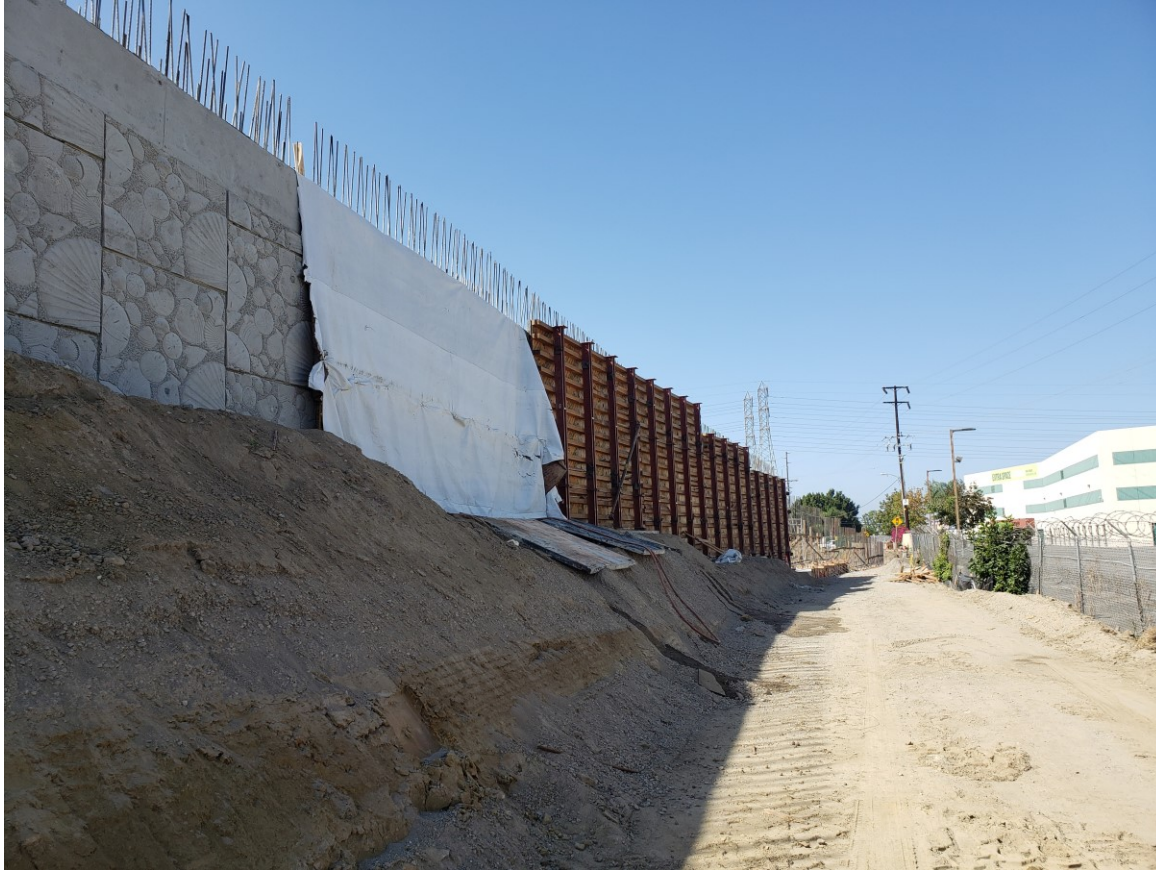
Retaining wall and soundwall construction
