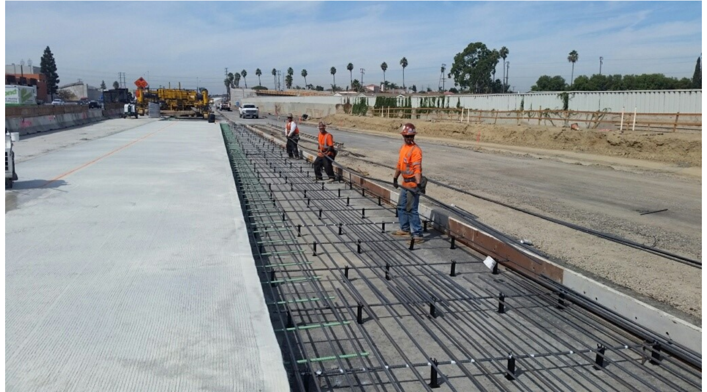
Concrete paving operations
