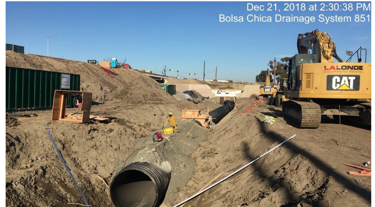
Bolsa Chica Road drainage system construction
