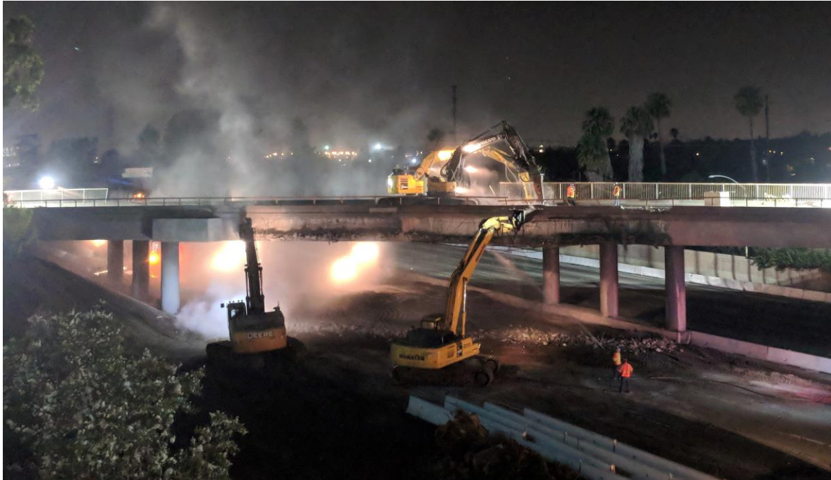
McFadden Avenue bridge demolition
