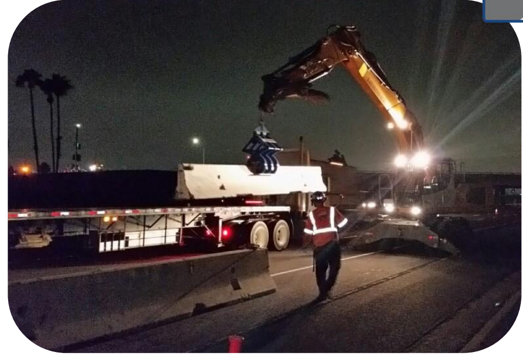
Placing k-rail
