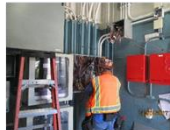
SA Hydrogen Gas Detection Control Panel Wiring
