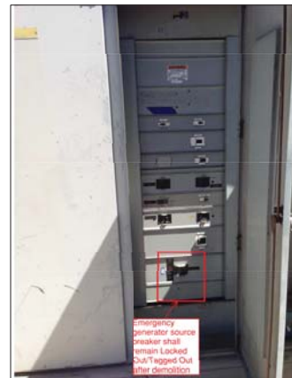
C EMERGENCY GENERATOR BREAKER CG-117 SCALE: NOT TO SCALE
