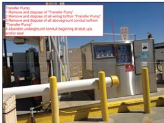
(A) TRANSFER PUMP SCALE: NOT TO SCALE
