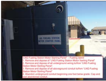
A MOTOR STARTER PANEL SCALE: NOT TO SCALE
