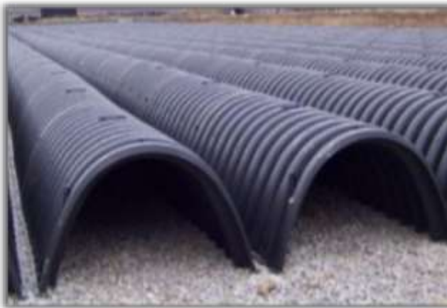
Underground Infiltration / Infiltration Gallery
