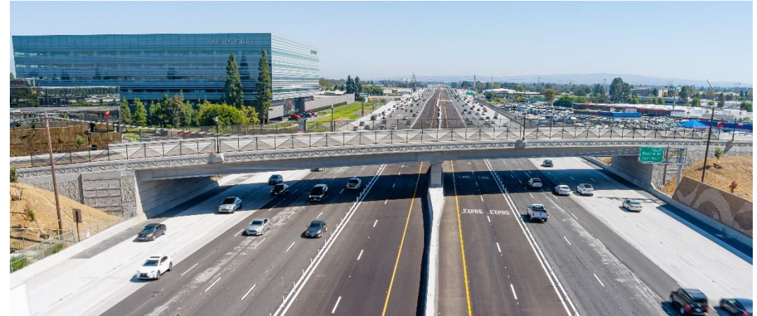
Ward Street bridge
