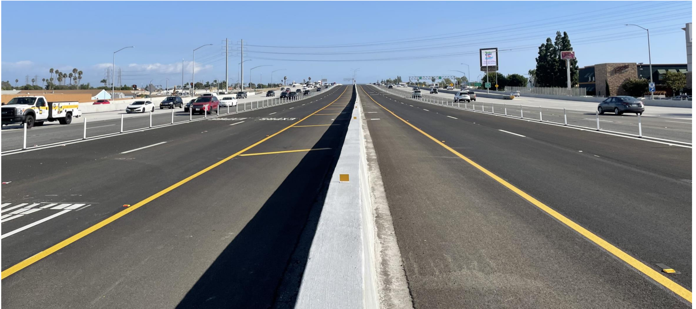
405 Express Lanes striping and channelizers
