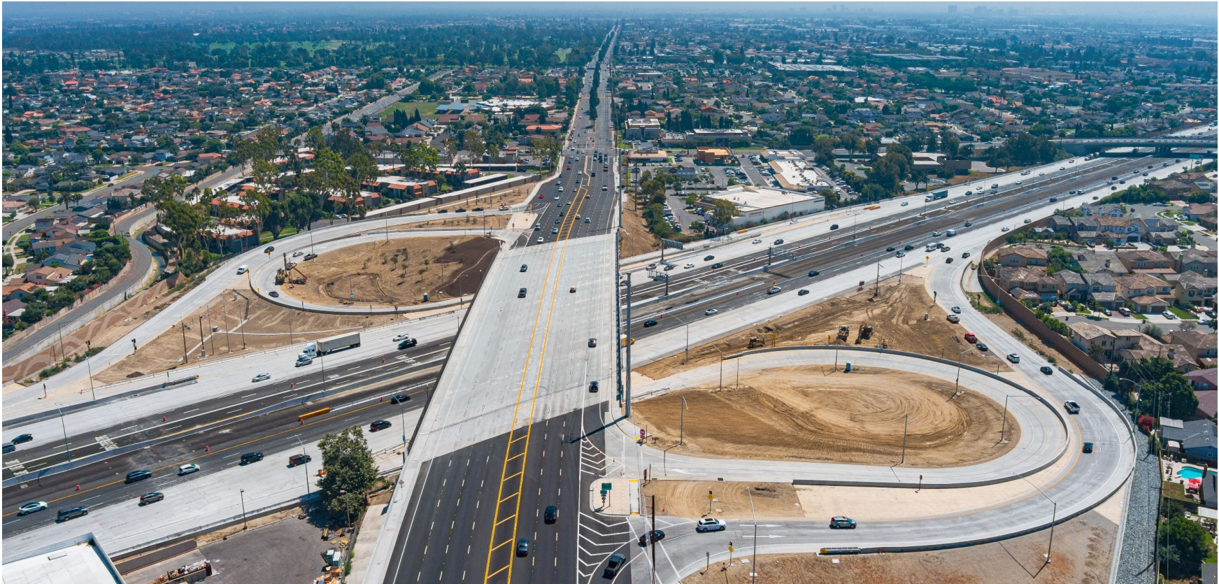
Warner Avenue bridge complete
