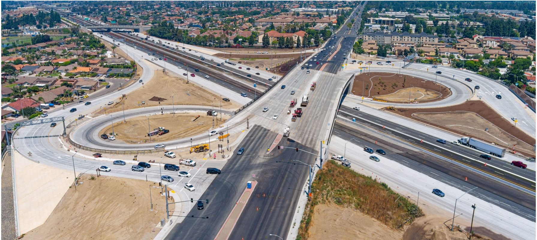
Brookhurst Street bridge complete
