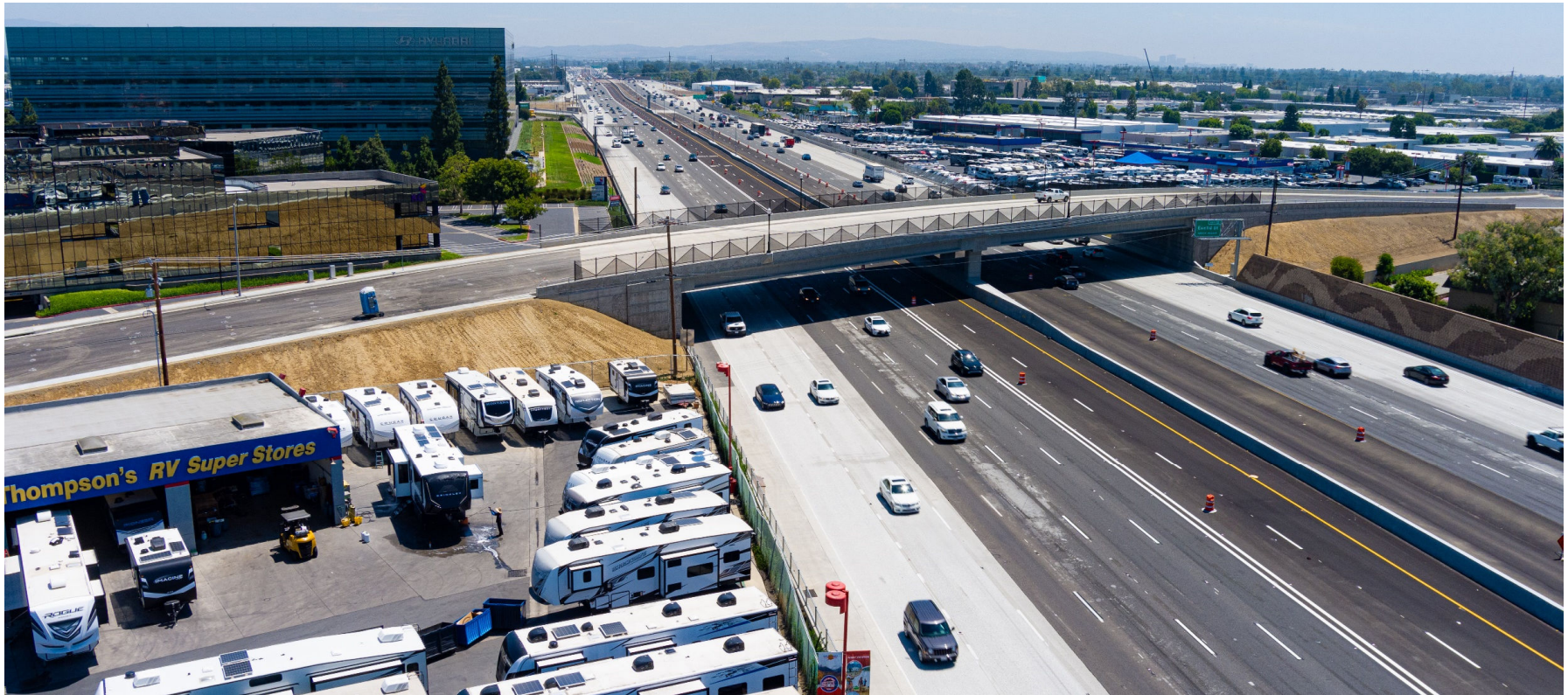
Ward Street bridge complete
