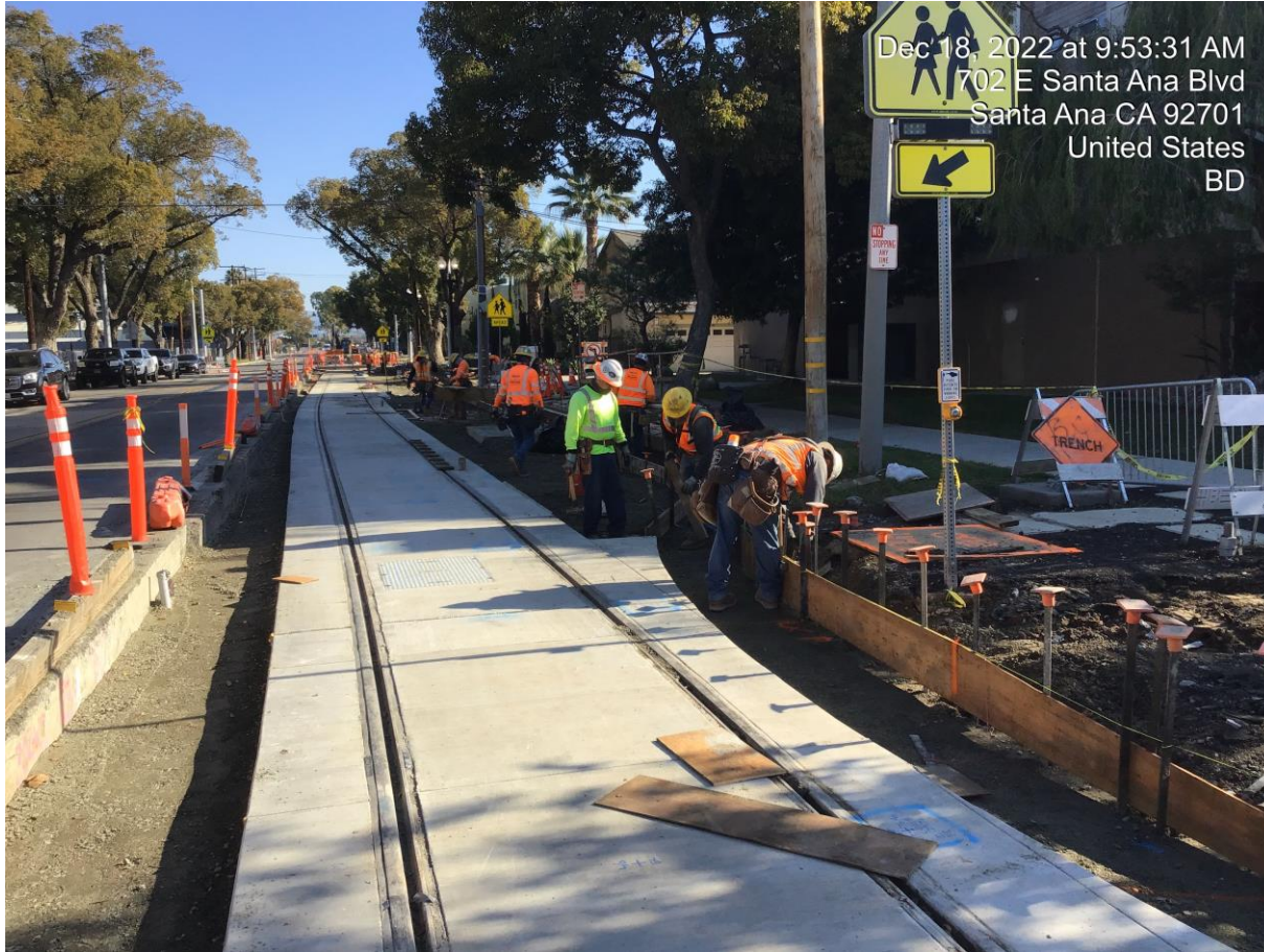
Embedded Track – Near Garfield Street
