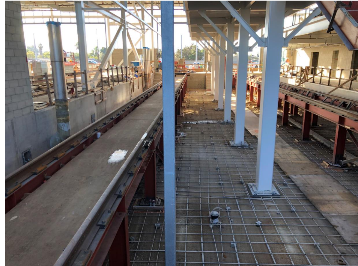
Tracks within the Service and Inspection Pit
