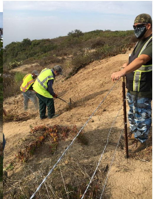
Breaking up large bike jump area. Workers pulled out over a dozen bags of dirt that formed the jump. Ground was left loose, broken up and dead brush was placed in the area. Site was monitored by Native American and archaeological contractors due to the proximity to sensitive resources. No cultural resources were detected.
