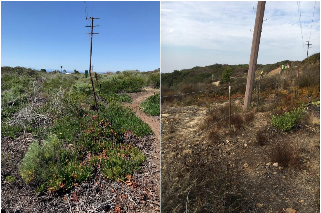
(Left) Old rusty barbed wire fence line. (Right) New smooth wire fence line (wildlife friendly). Contractor was able to utilize some of the same posts. Fence is in the same location.
