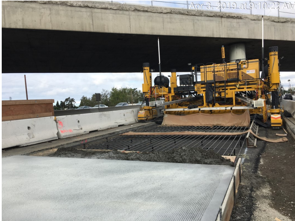
Concrete paving operations
