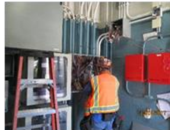
SA Hydrogen Gas Detection Control Panel Wiring
