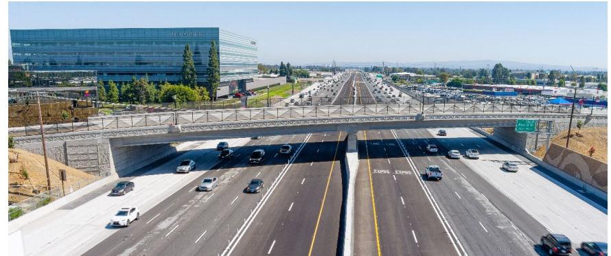
Ward Street bridge
