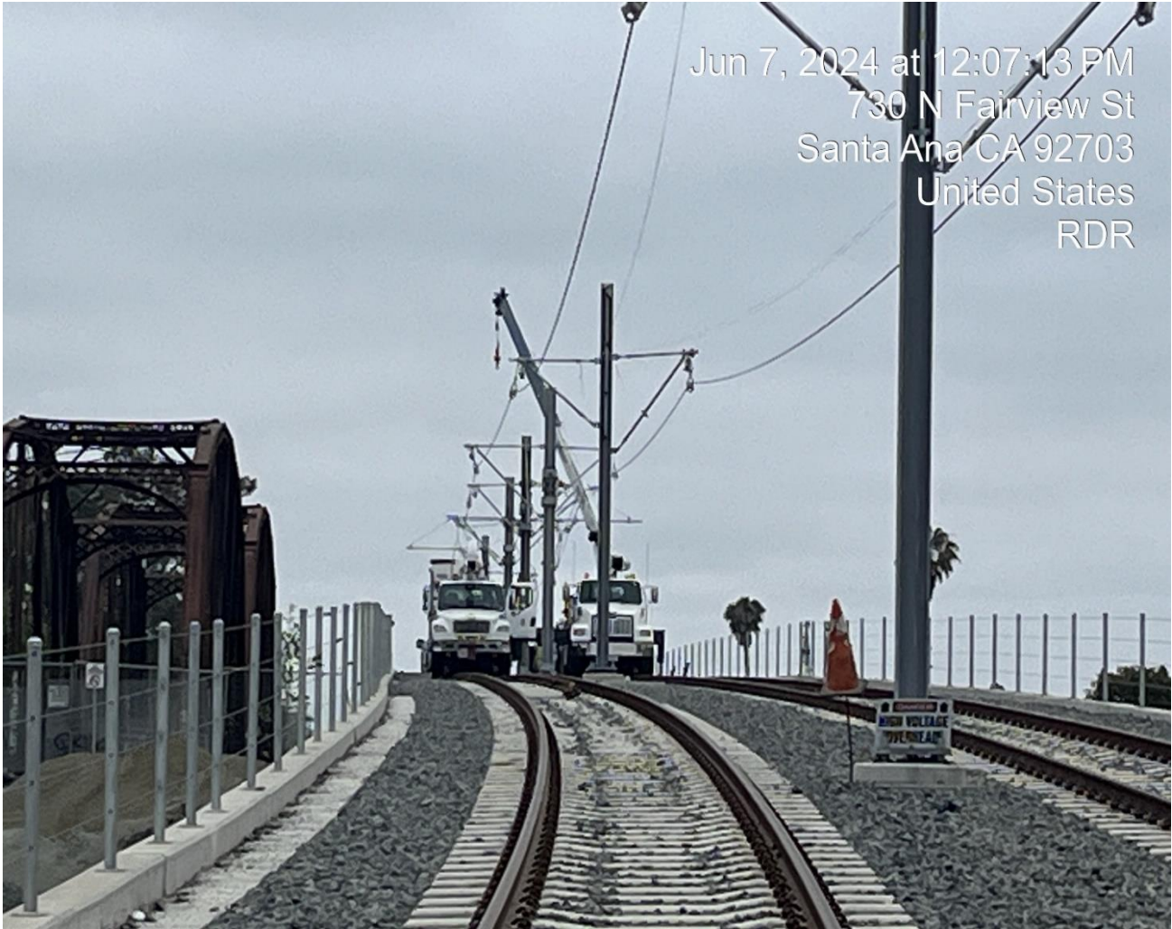
OCS Wire Installation
