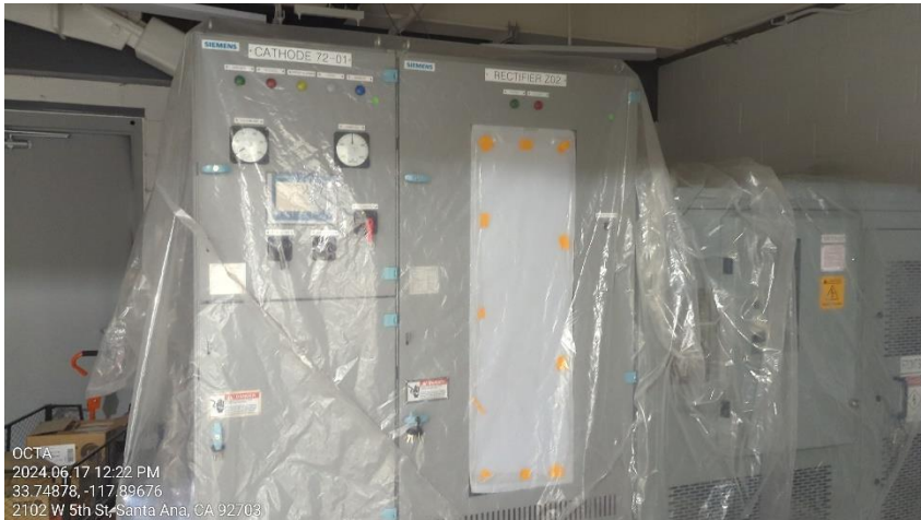
Control gear installation
