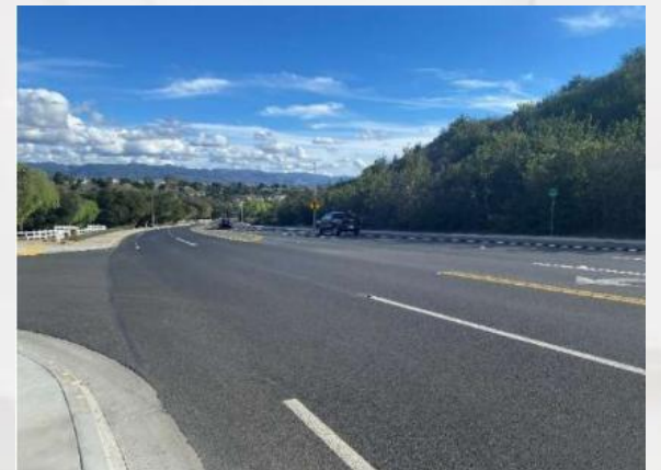
Wagon Wheel Pavement Rehabilitation Overlay Project
