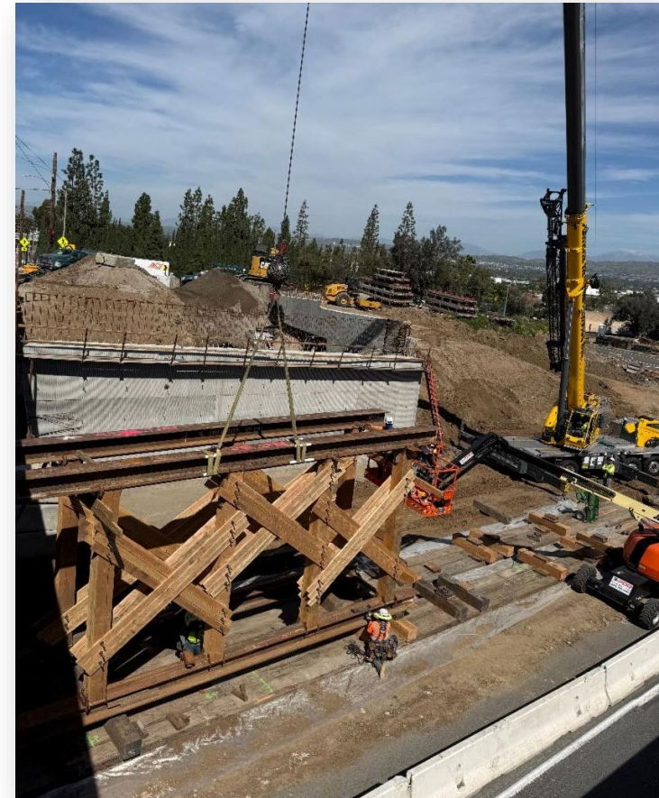
Placement of temporary support structures for the Lakeview Avenue bridge
