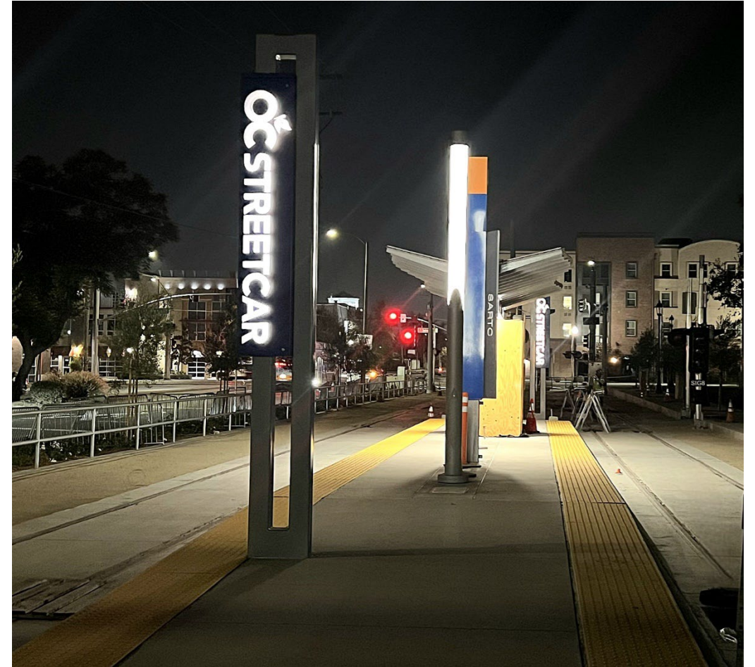
Energized Santa Ana Regional Transportation Center Platform
