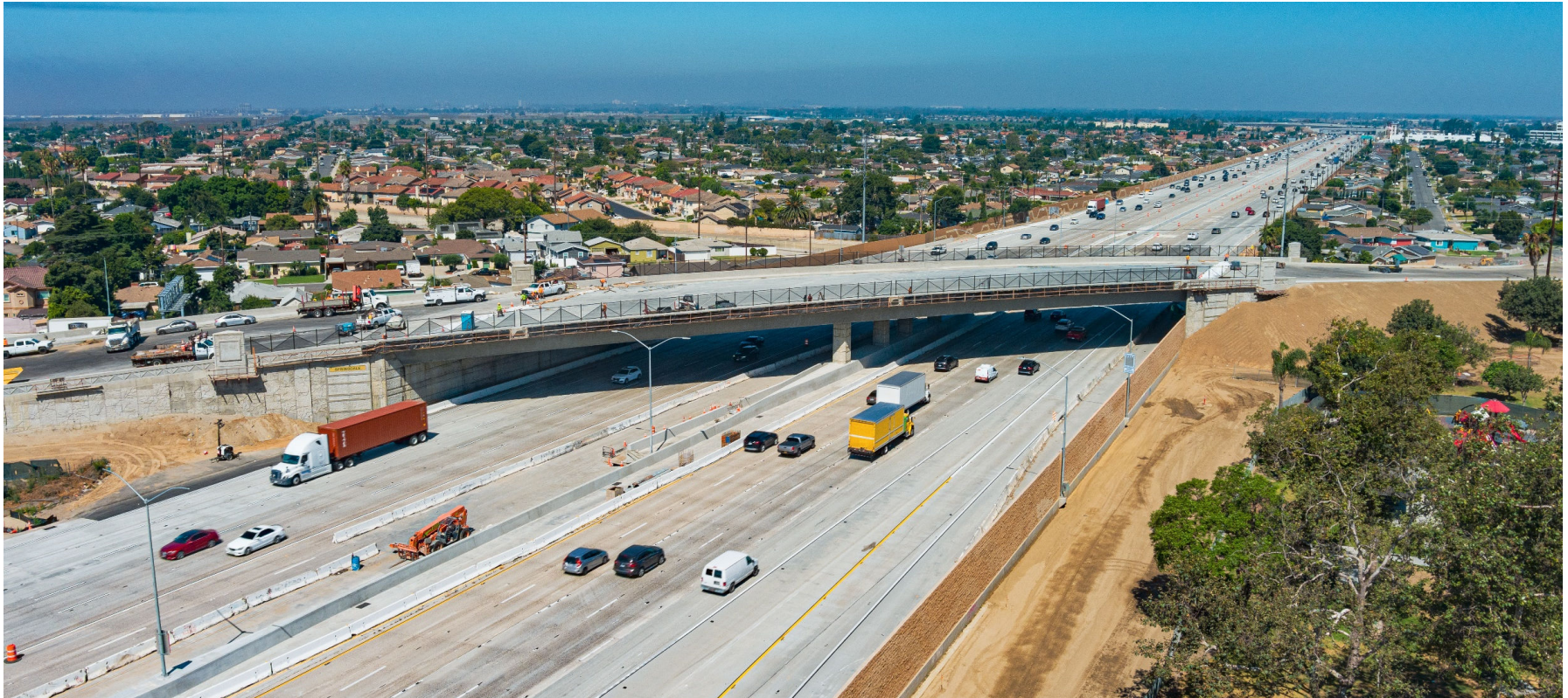
Springdale Street bridge complete
