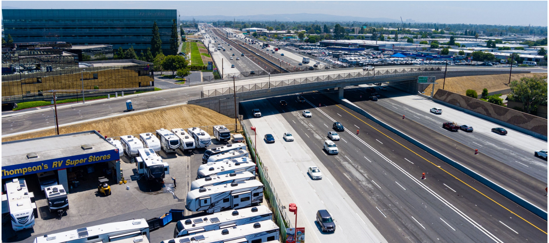
Ward Street bridge complete
