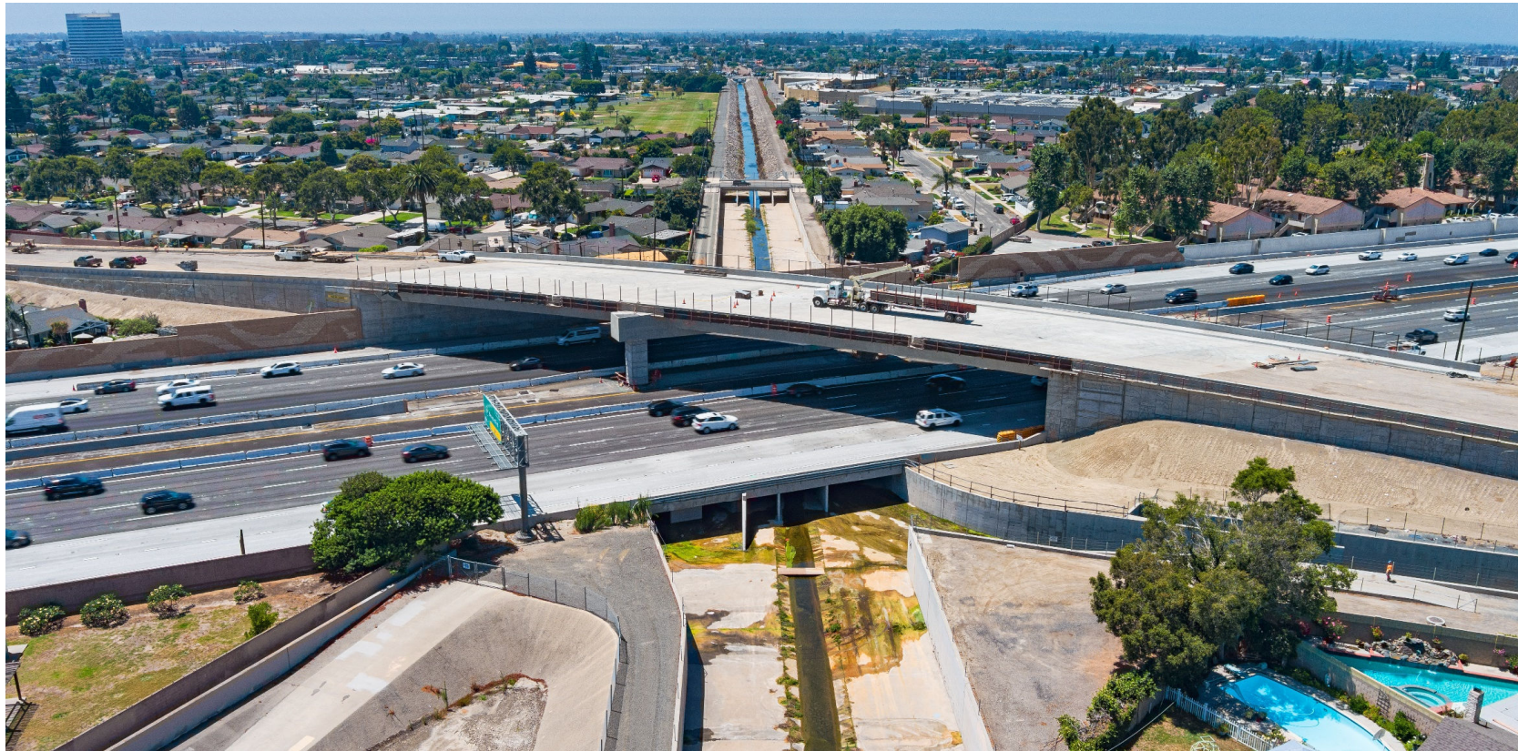
Newland Street bridge complete
