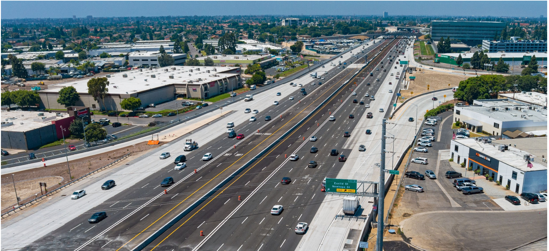
Express Lanes striping
