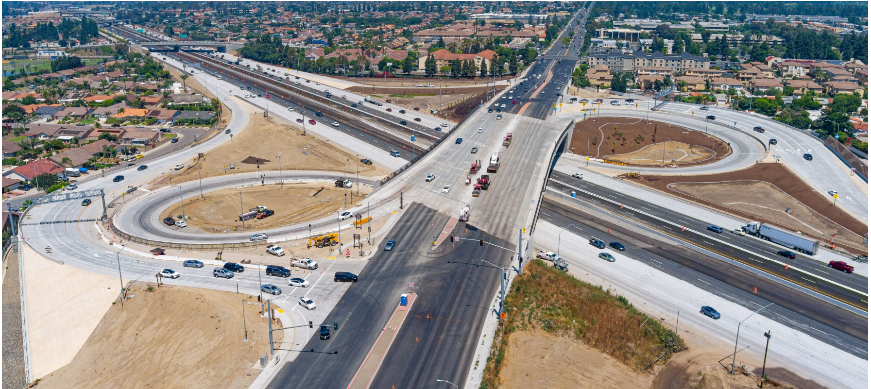
Brookhurst Street bridge complete
