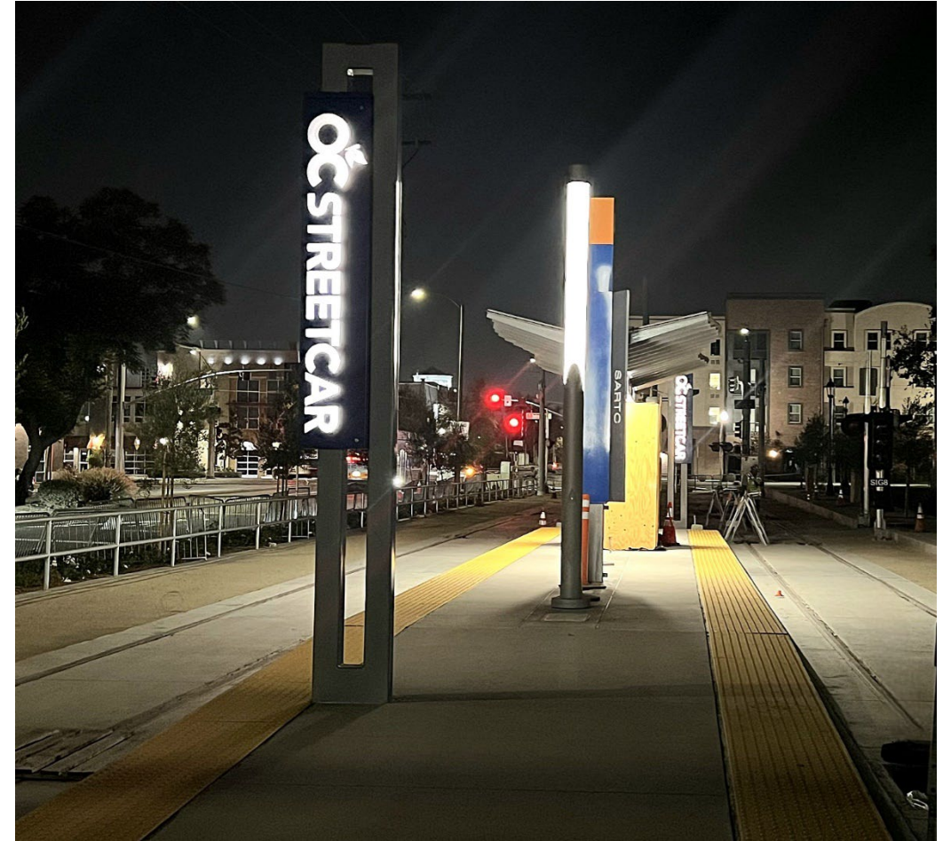
Energized Santa Ana Regional Transportation Center Platform
