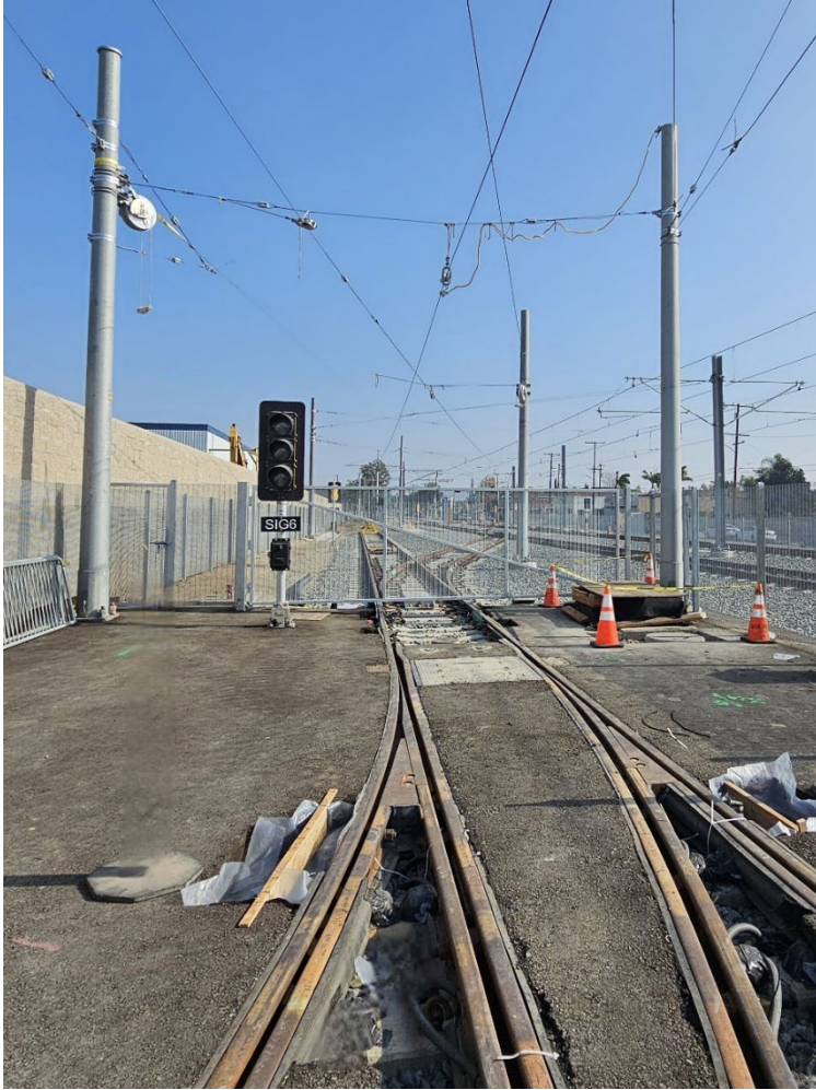
Installed Gate and Overhead Contact System (OCS) Wire
