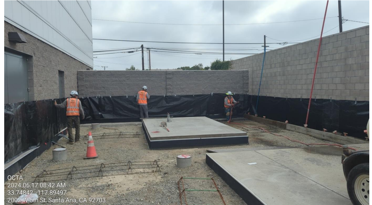
Generator pad preparation
