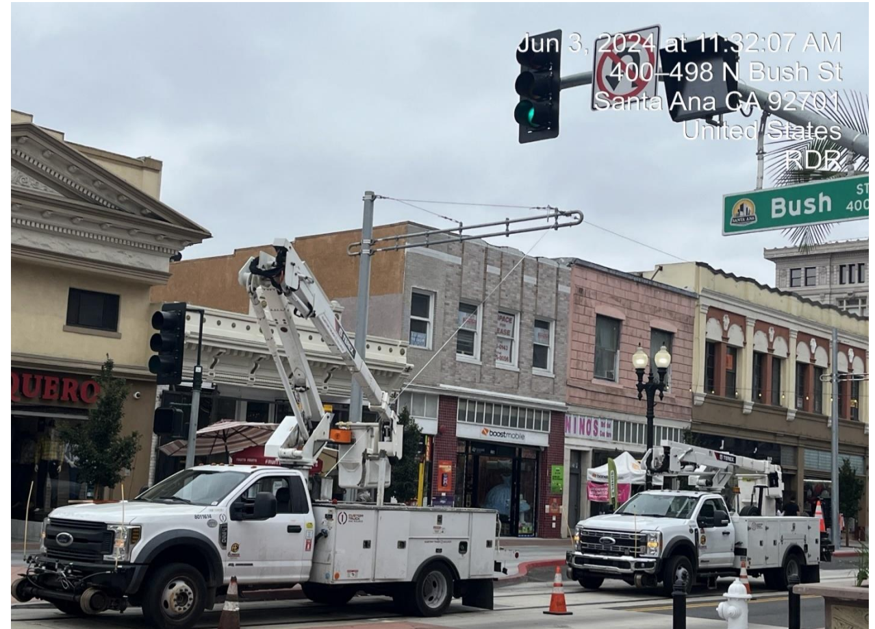
Installation of OCS Bracket Arms
