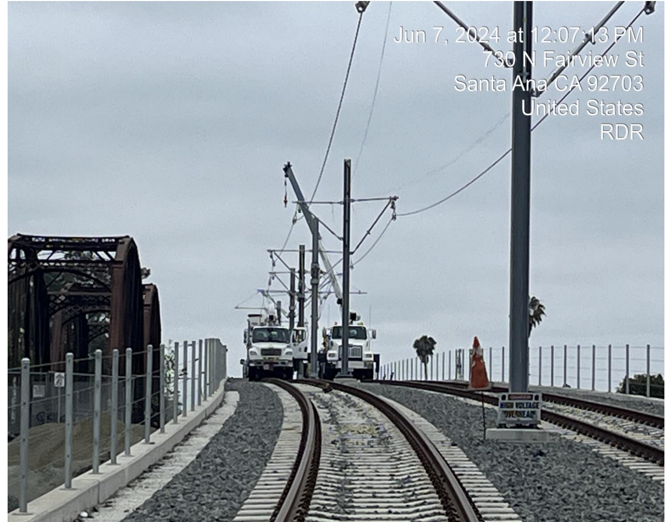
OCS Wire Installation
