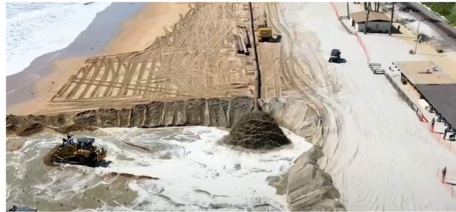
Pictures from San Clemente Sand Replenishment Project
