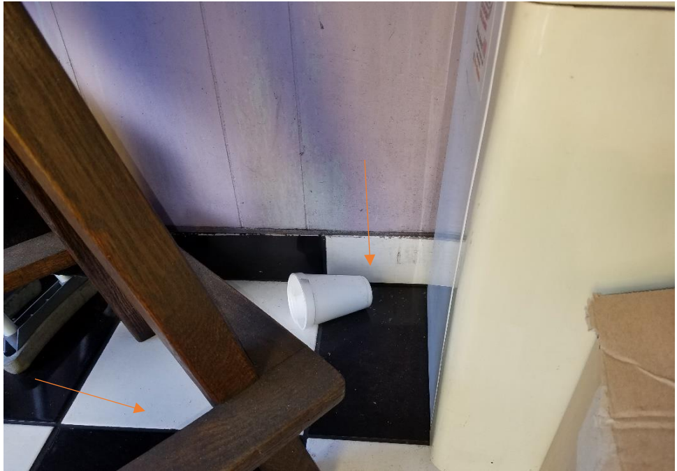
Photograph 7: View of the lead-containing white ceramic wall tile and baseboard in Unit 1516 office.
