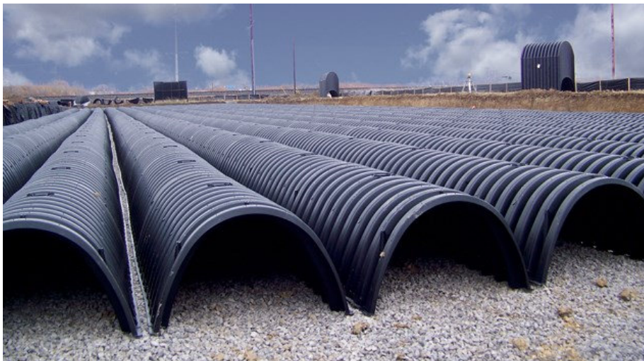
Figure 2.3.3 – Typical Underground Infiltration Chambers
