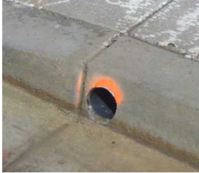
Figure 2.3.2 – Typical Roof Drain Curb Outlet at Sidewalk
