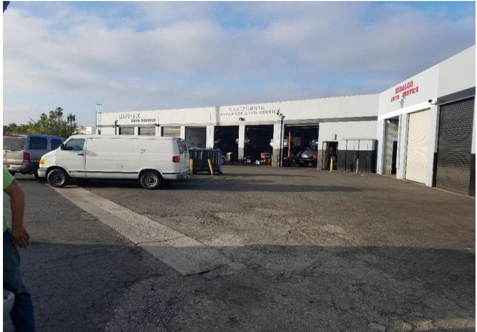
Photograph 1: General view of the site structure.
