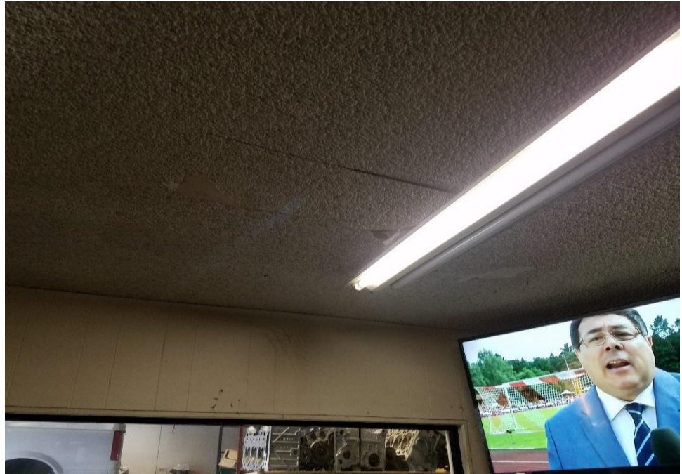
Photograph 11: View of representative fluorescent lights and ballasts.
