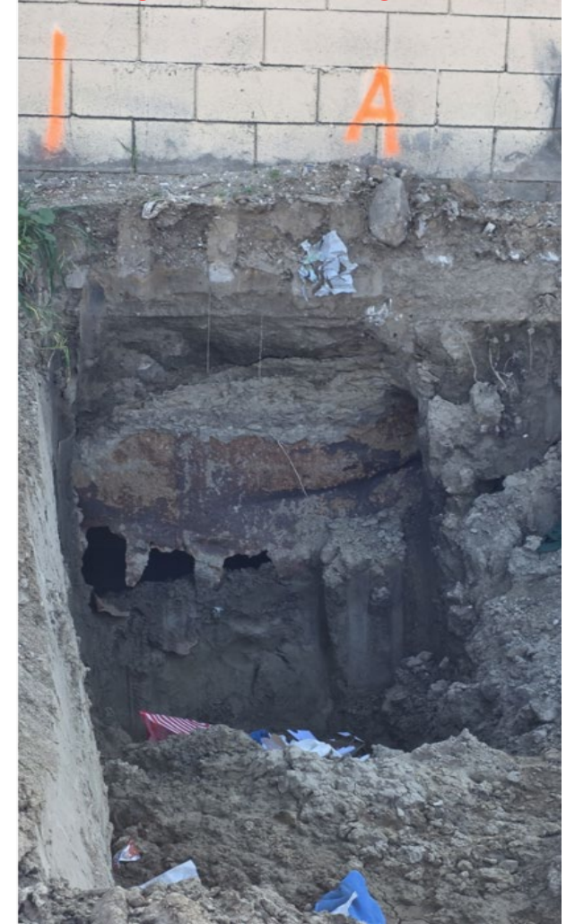
Underground storage tank 2
