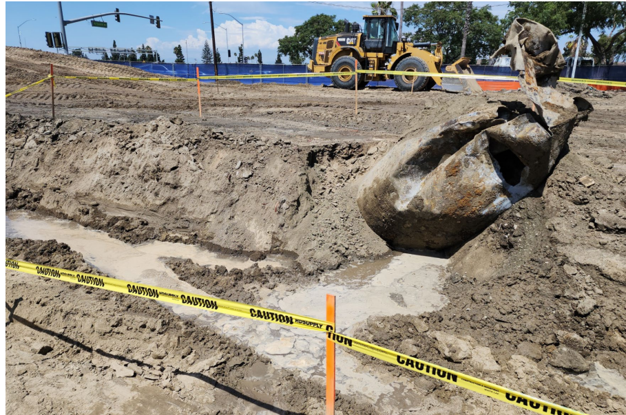
Underground storage tank (UST) 1
