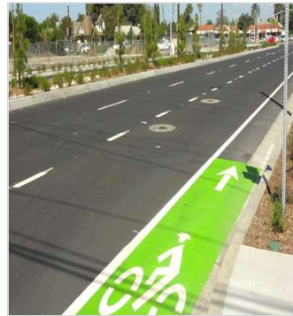
Grand Avenue Improvements City of Santa Ana
