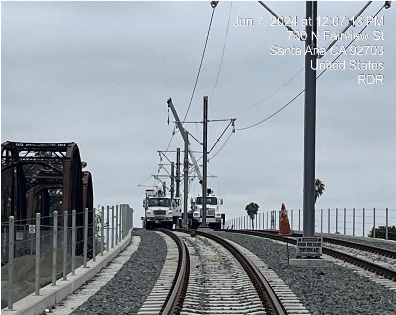
OCS Wire Installation
