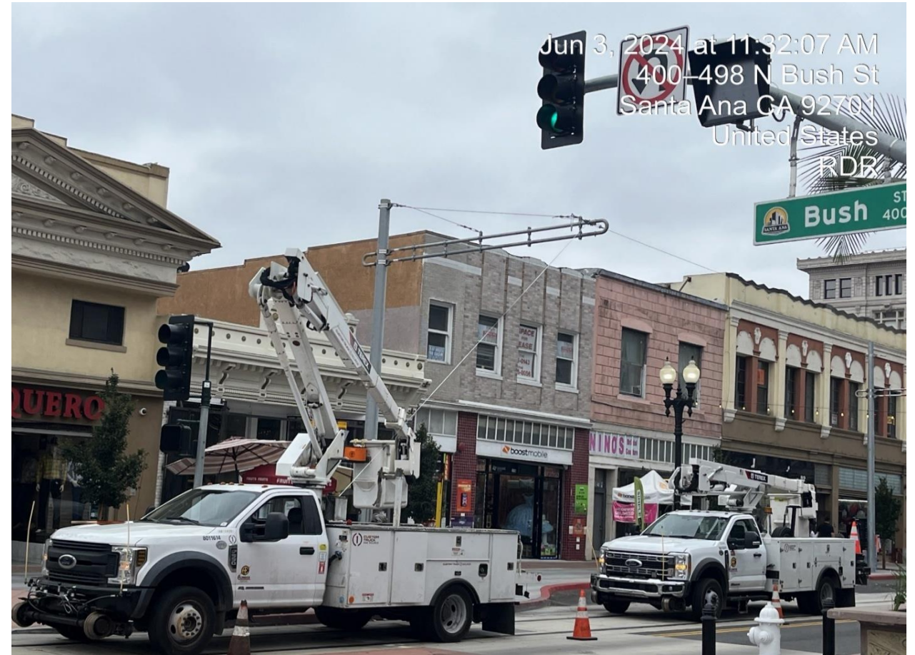
Installation of OCS Bracket Arms
