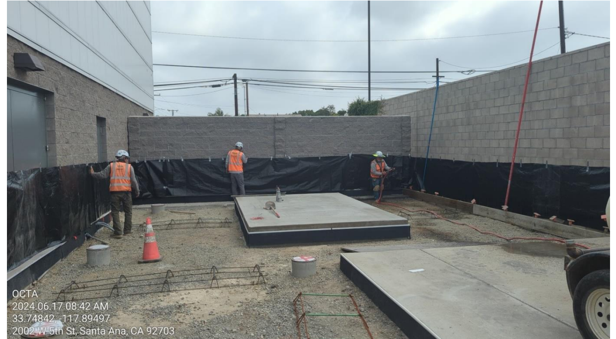
Generator pad preparation
