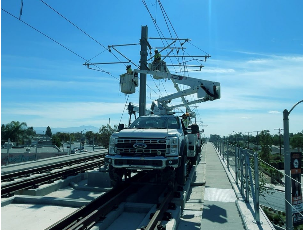
Overhead Contact System (OCS) Wire Installation
