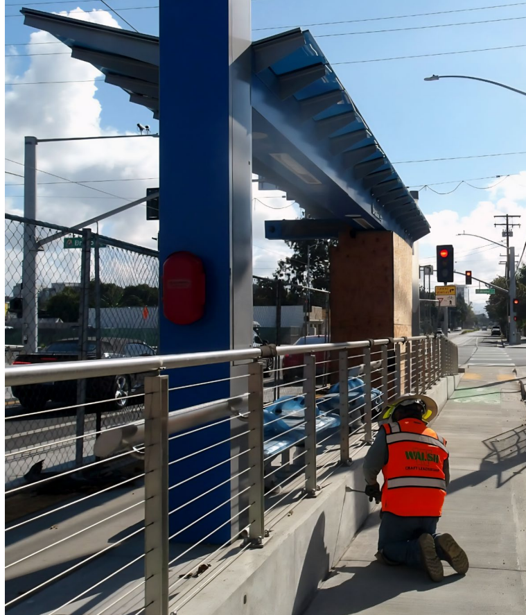
Bristol Street platform punchlist work
