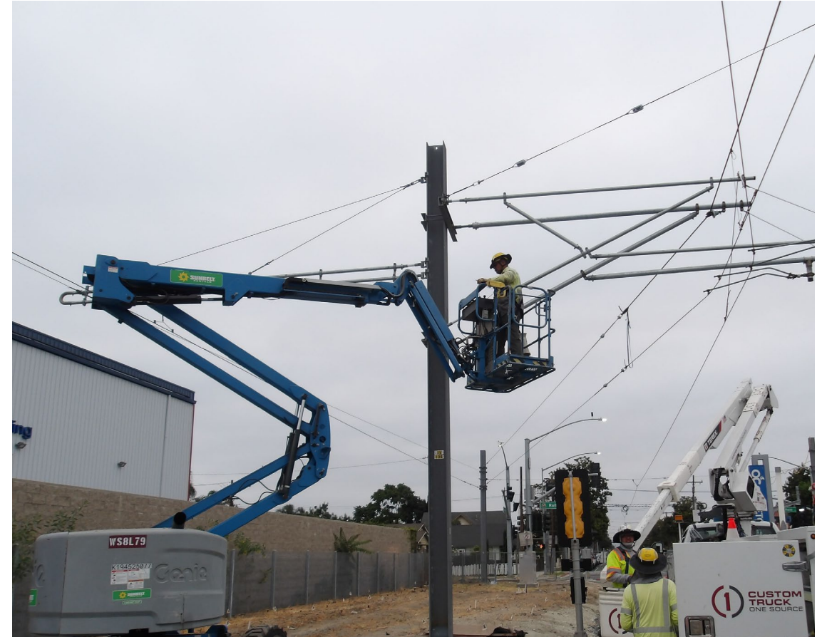
Overhead Contact System (OCS) Wire Installation
