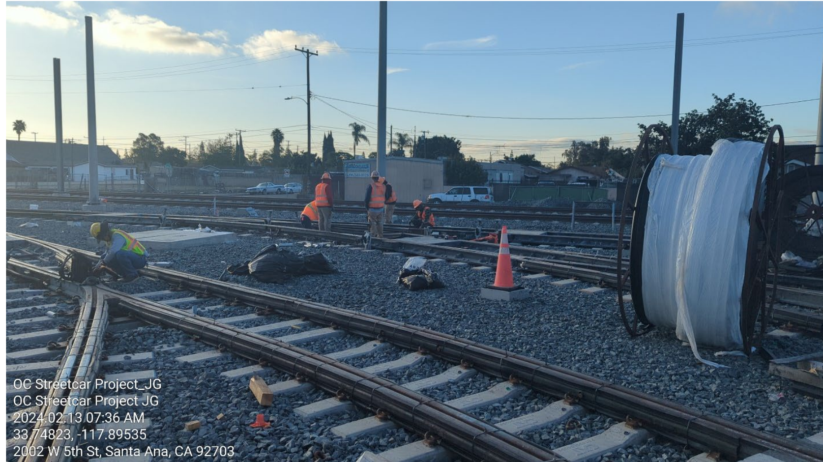
Preparation for paving for the yard track
