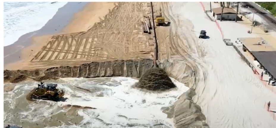
Pictures from San Clemente Sand Replenishment Project
