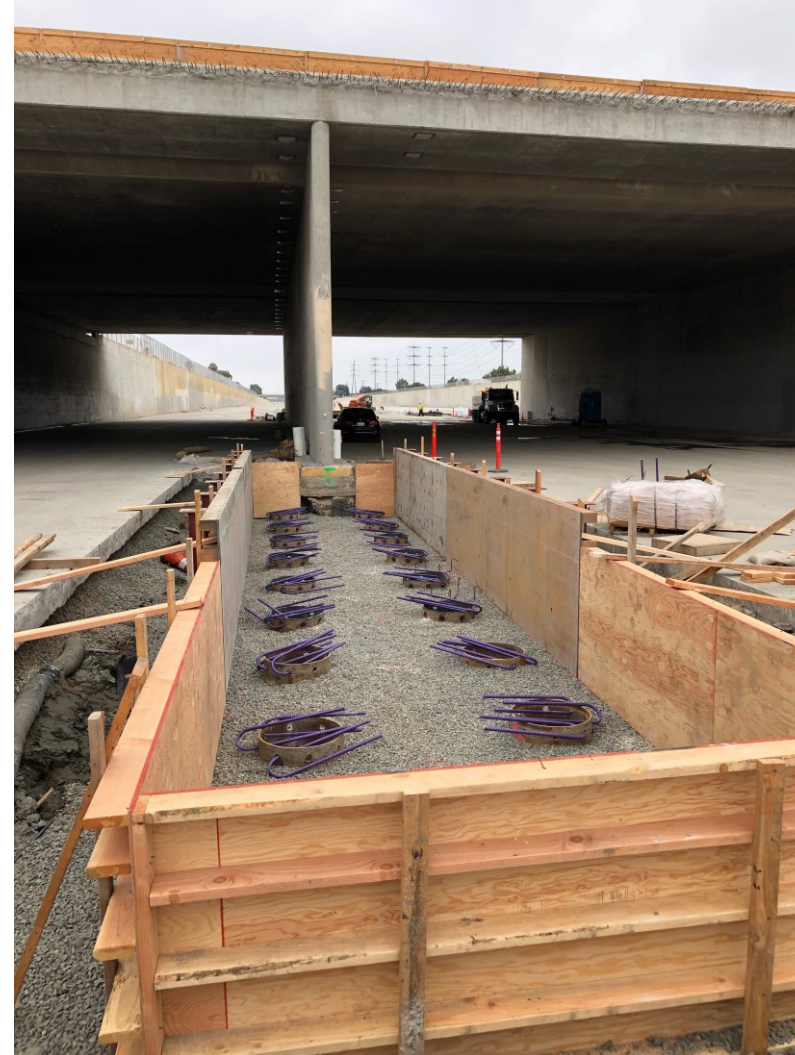
Santa Ana River bridge construction
