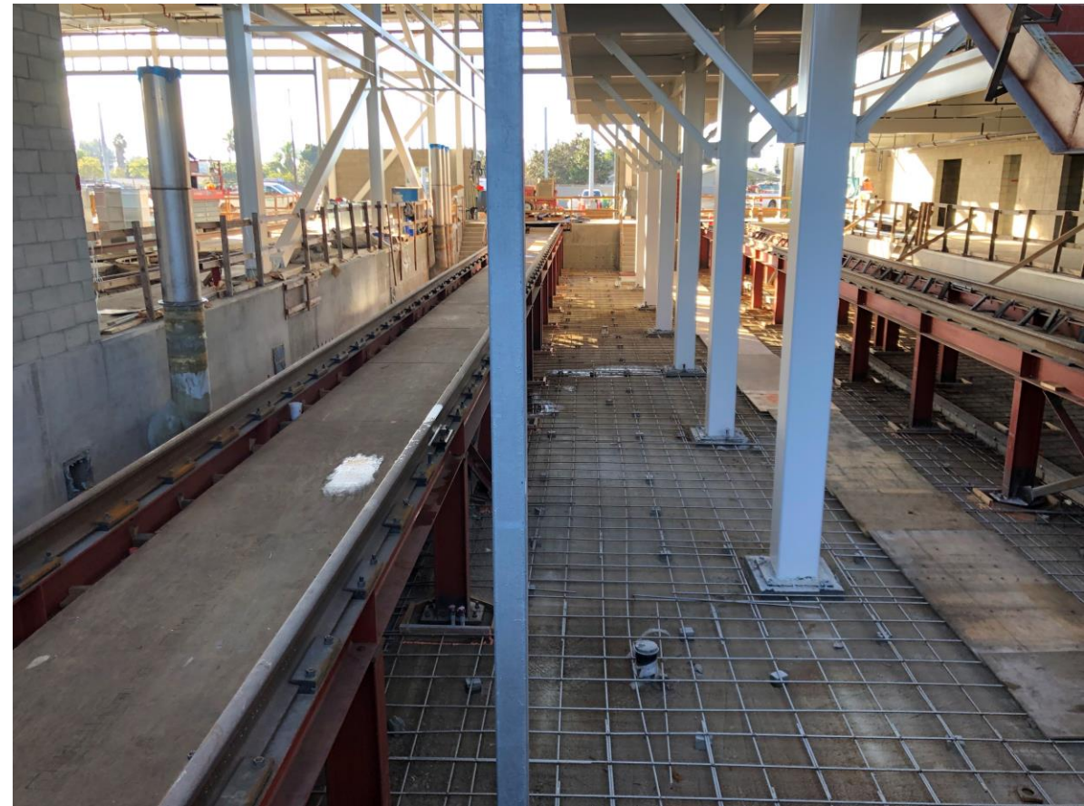
Tracks within the Service and Inspection Pit
