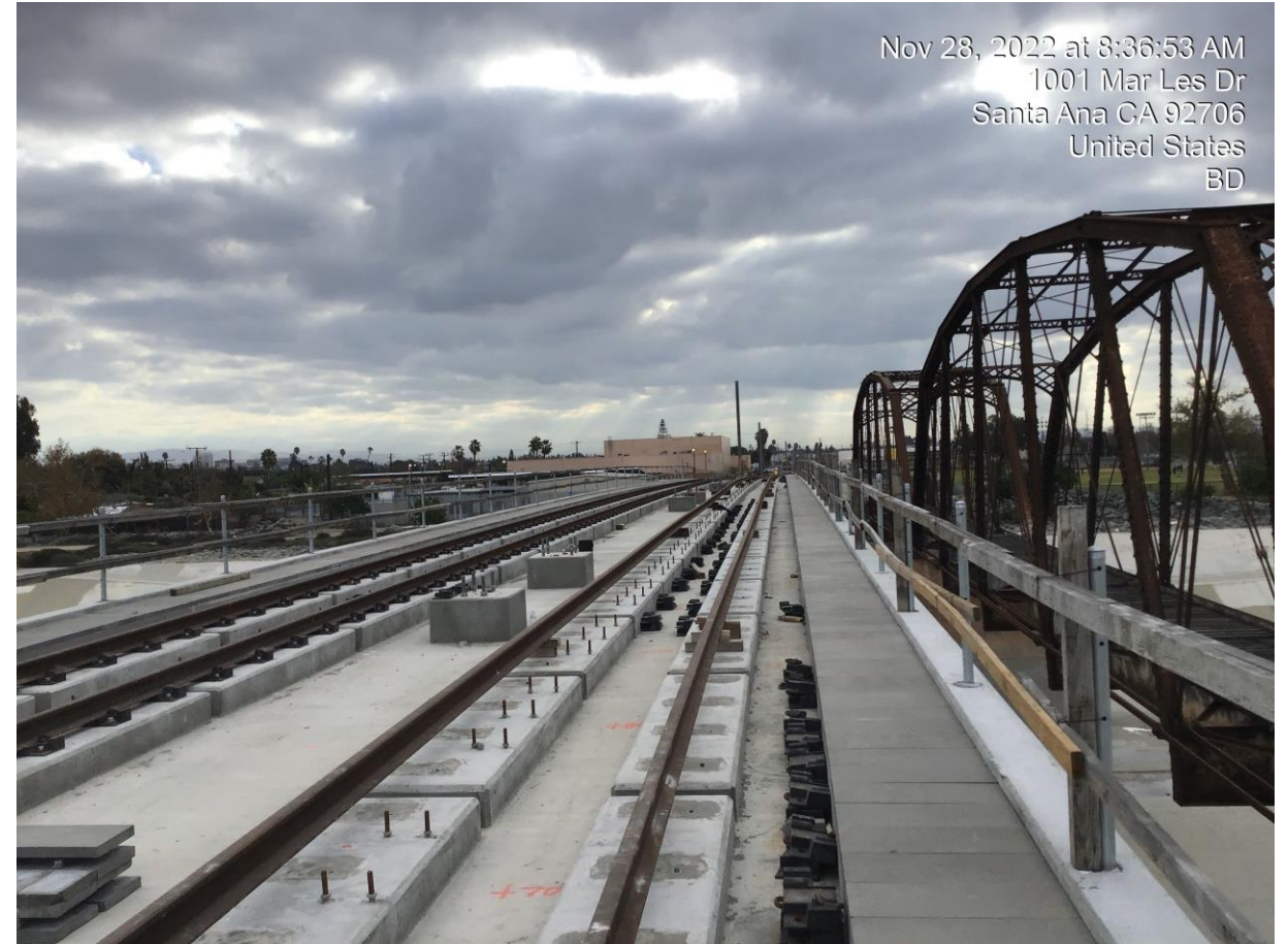
Santa Ana River Bridge Plinths
