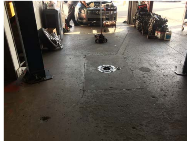
Photograph 5. View of one of the decommissioned in-ground hoists beneath the above ground hoist in the California Japanese Auto Service unit.
