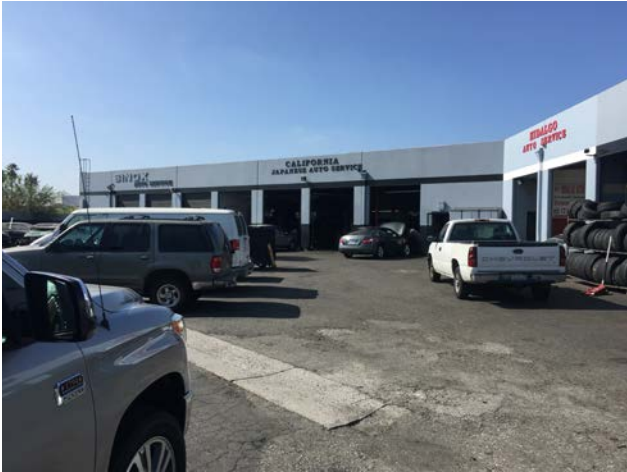
Photograph 1. View of the onsite structure, facing south.
