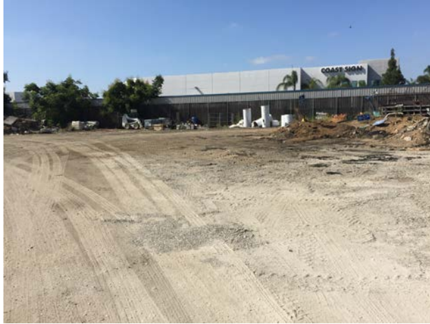
Photograph 14. View of storage on the southern portion of the site, behind the locked gate, facing south.
