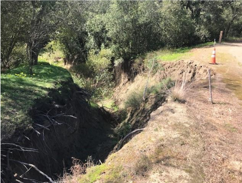
Gully – Before Construction of Phase 1 (March 2021)
