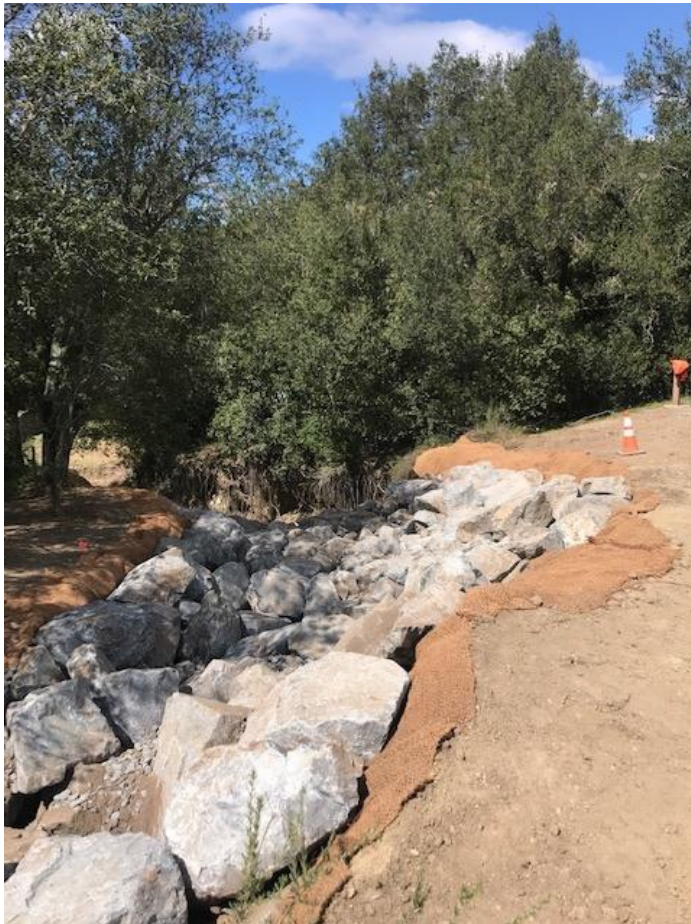
Gully – Post Construction of Phase 1 (April 27, 2021)
