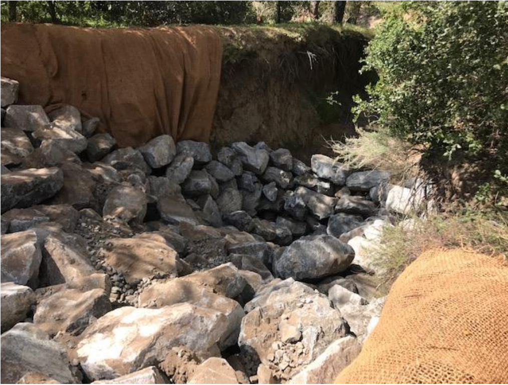
Trabuco Rose Gully Photos April 2021
