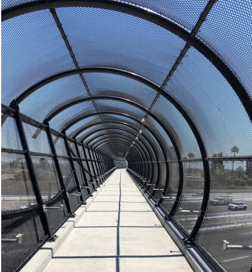
Heil Avenue (pedestrian) bridge construction
