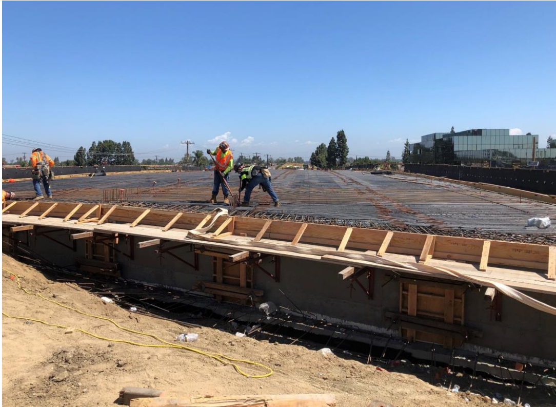
Ward Street bridge construction
