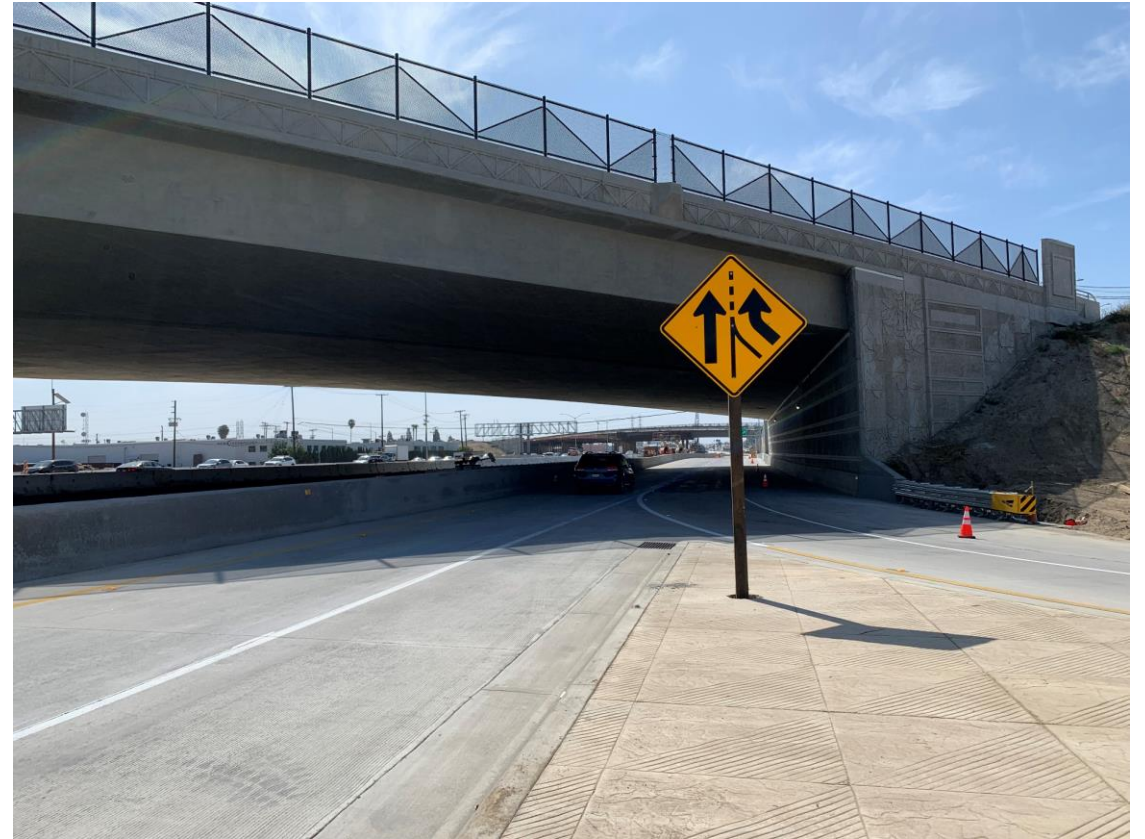
Goldenwest Street bridge construction
