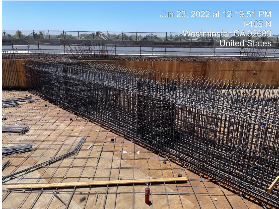
Bolsa Avenue bridge construction
