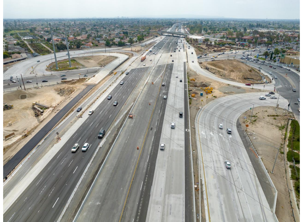
Beach Boulevard construction
