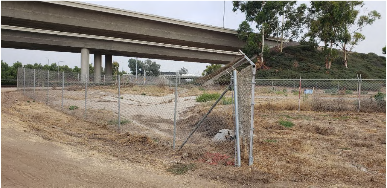
Photo 9 A bridge carrying rail tracks into the site from rail tracks visible in the background would cross over this portion of the Bee Canyon channel.
