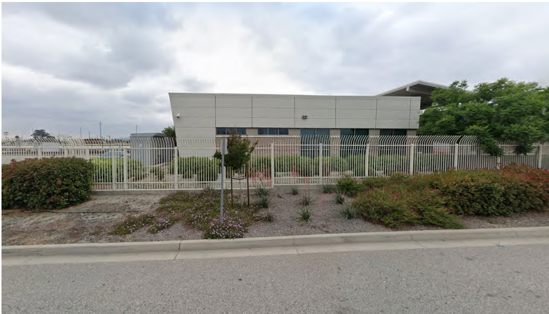
Figure 5.4-2 Existing Eastern Maintenance Facility, Exterior Building Materials
