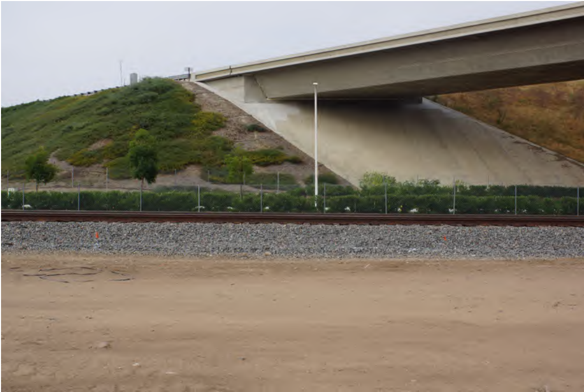
Figure 3.3.5-2 Overview of P-30-176663, Former AT&SF Railroad from Project APE, View to West
