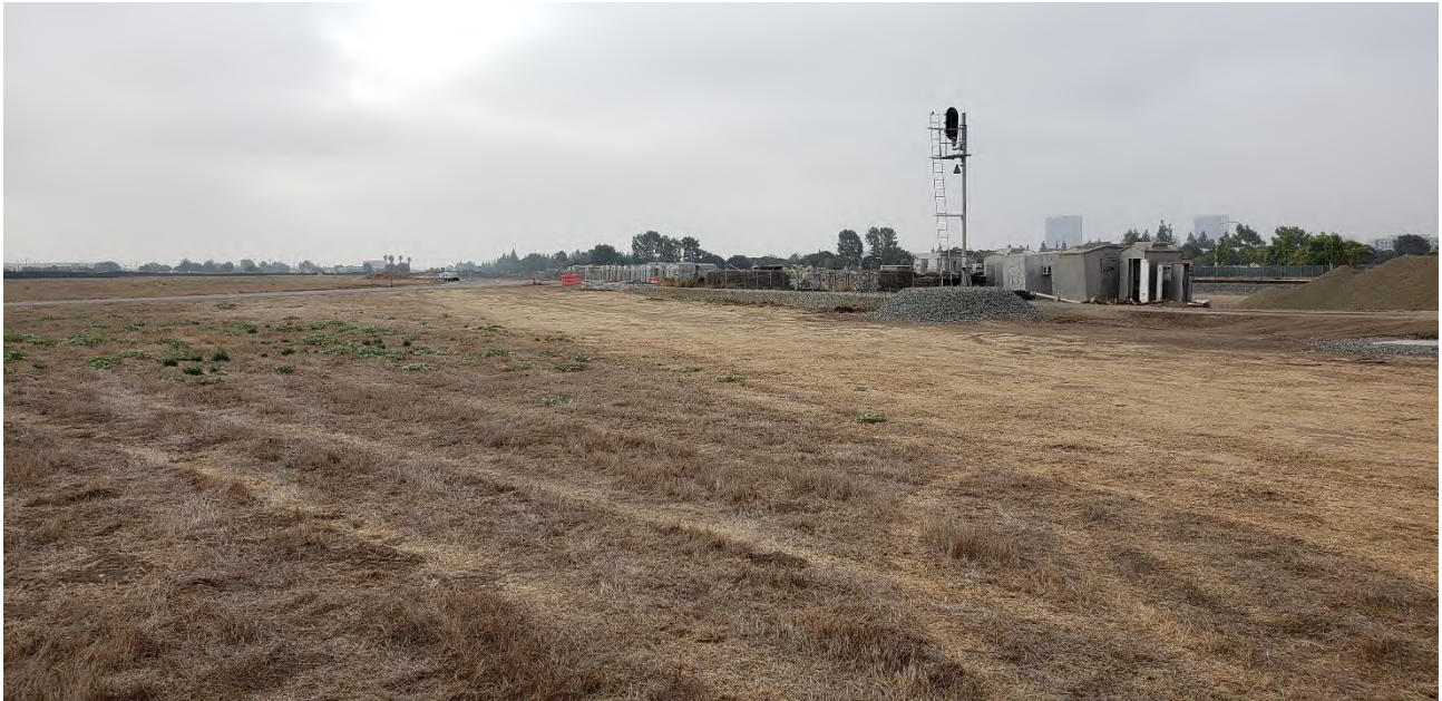
Photo 1. Southeast-facing view from the northwest corner across Project Site. Marine Way is visible at left, with miscellaneous rail equipment and materials stored onsite and rail tracks at right.
