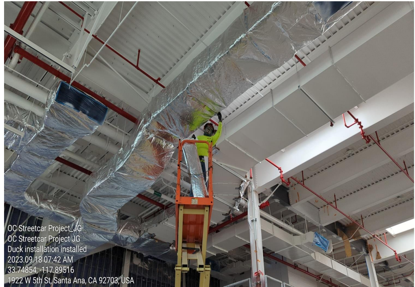
Installation of Duct Insulation
