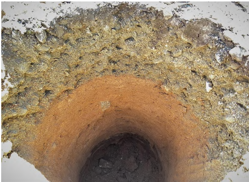
Figure 4. Soil profile at STP 3 showing deep layer of road base
