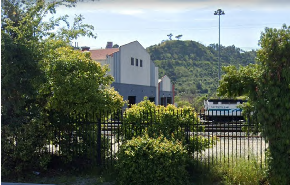
Figure 5.4-1 Existing Central Maintenance Facility, Exterior Building Materials
