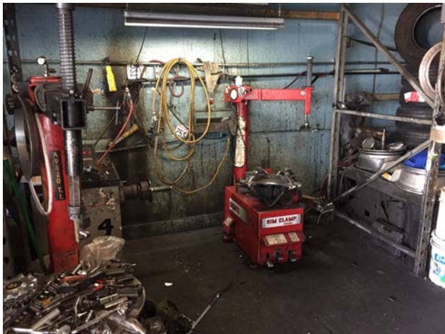
Photograph 10. View of the machinery area in the southern Yency's Tires unit.
