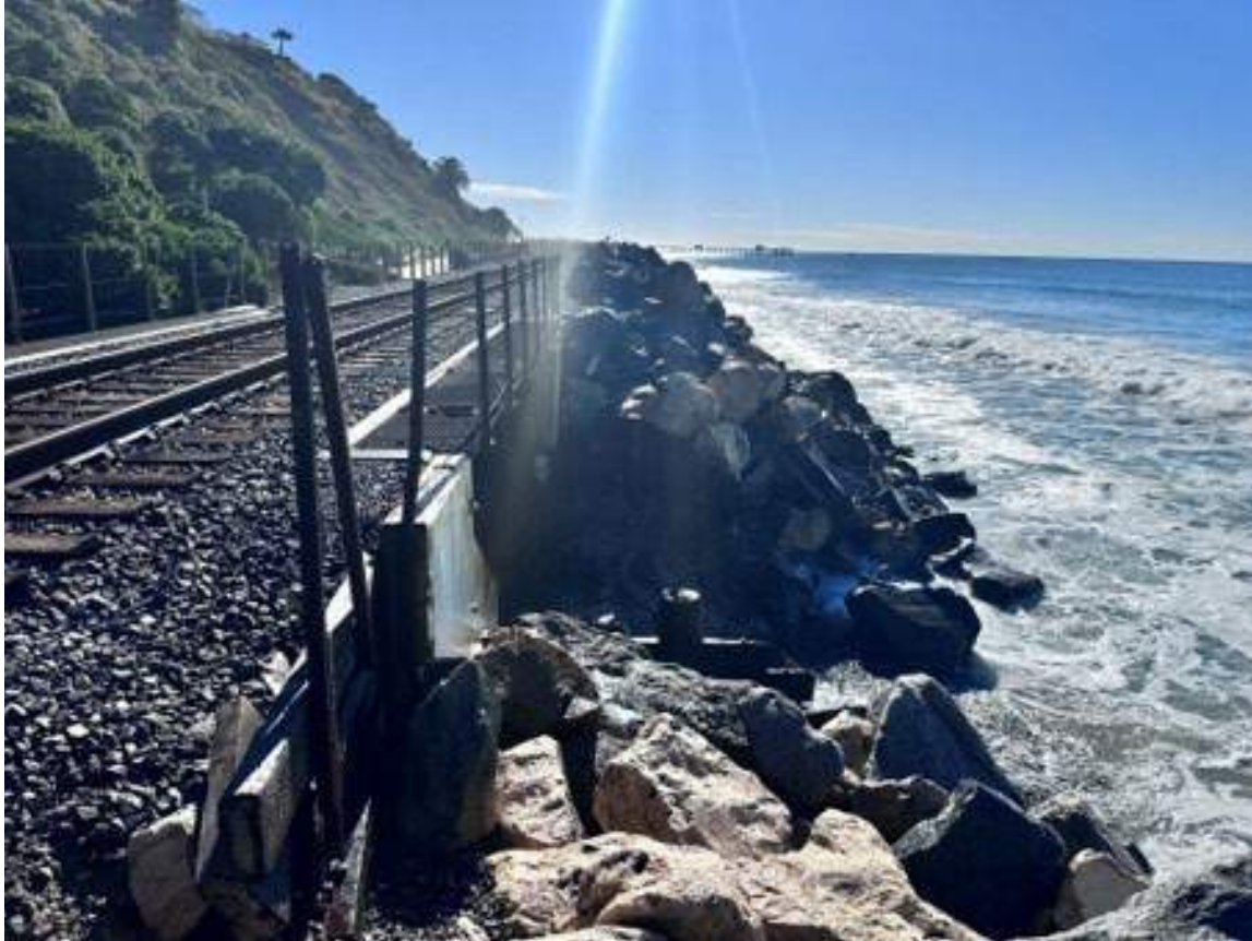
Figure 14. Potential Reinforcement Site 2: MP 204.10, November 2023
