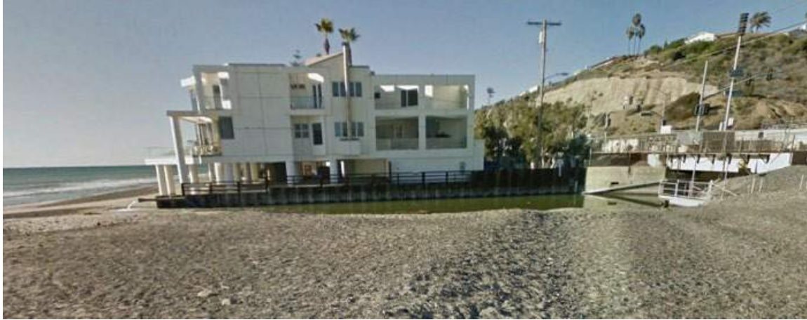
Figure 7. Monitoring Site 2: MP 202.70, Poche Beach Outfall and Pedestrian Underpass
