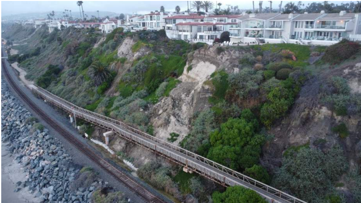
Figure 9. Monitoring Sites 4 and 5: MP 204.00–204.30, Mariposa Pedestrian Bridge – January 21, 2024.
