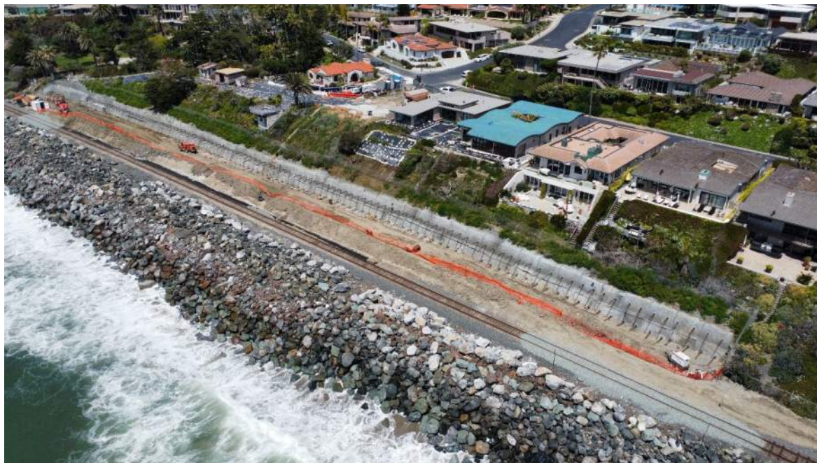
Figure 1 MP 206.80 Track Stabilization Project (Cyprus Shore) May 2023
