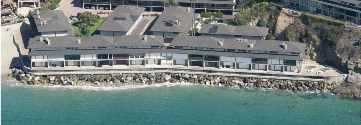
Figure 25. Combination Wall in Laguna Beach, CA
