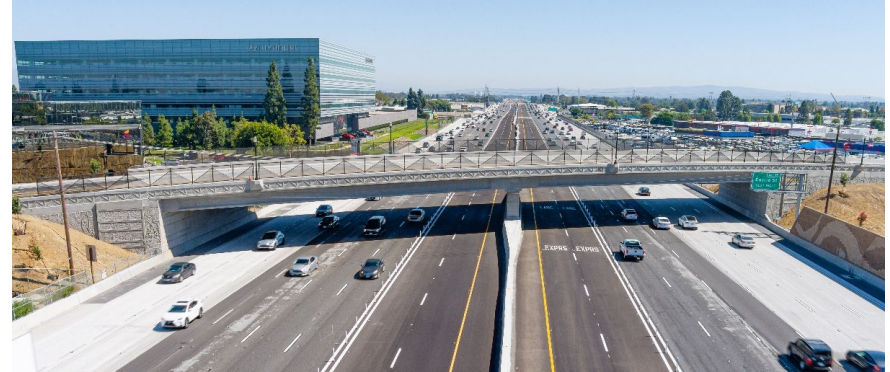
Ward Street bridge
