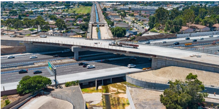
Newland Street bridge
