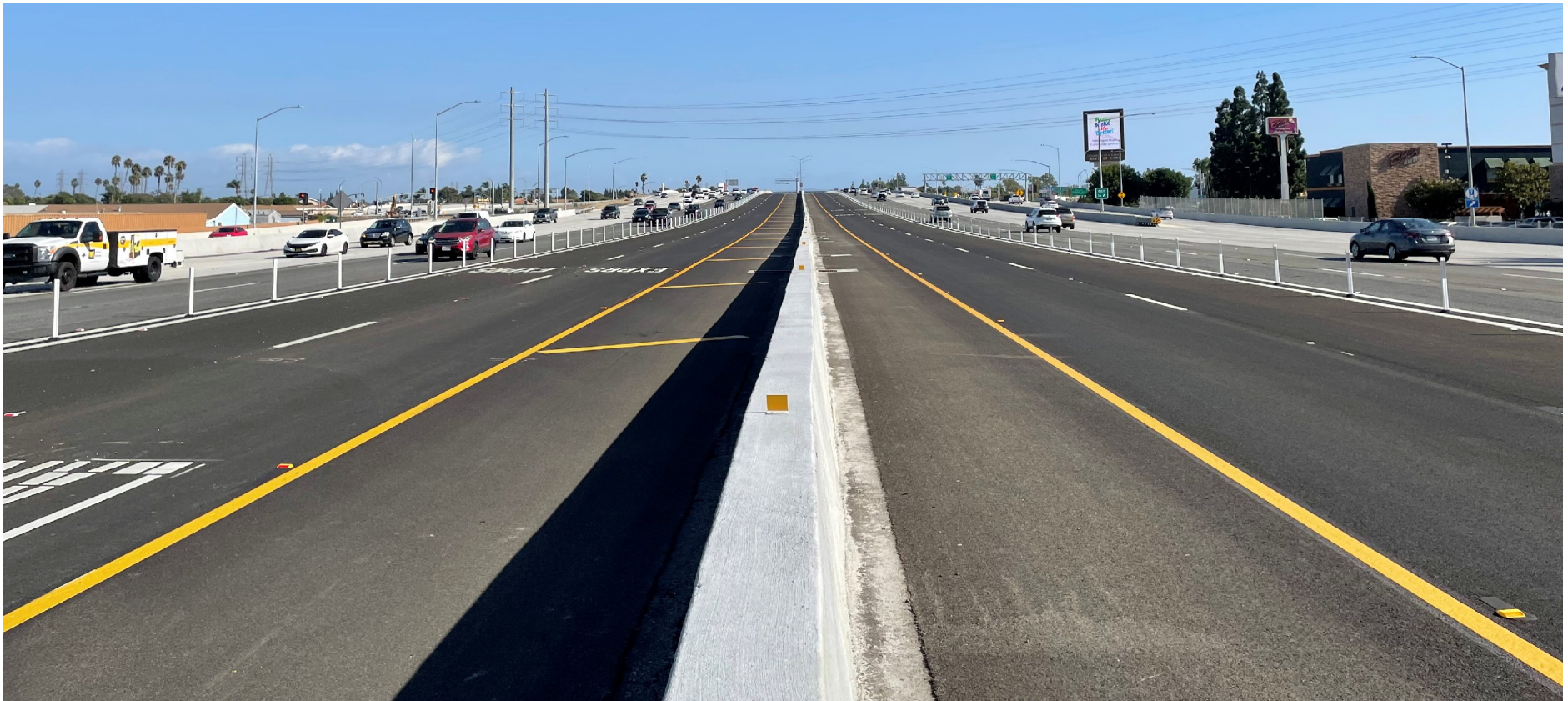
405 Express Lanes striping and channelizers
